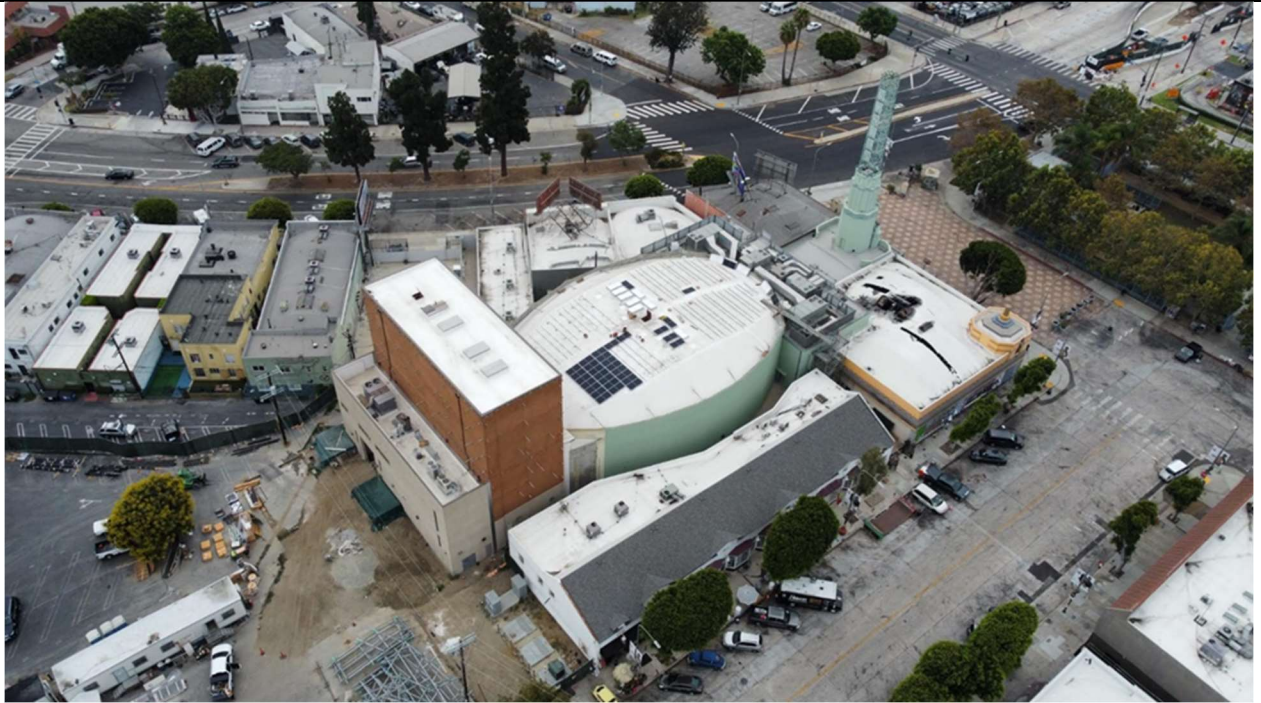
Aerial View of the Vision Theatre construction progress
