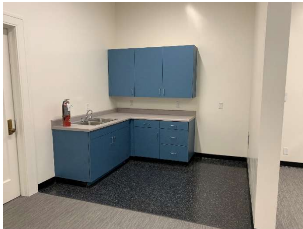
Figure 3 Kitchenette area from Phase 1.5
