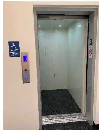
Figure 4 First floor lobby area and elevator from Phase 1.5
