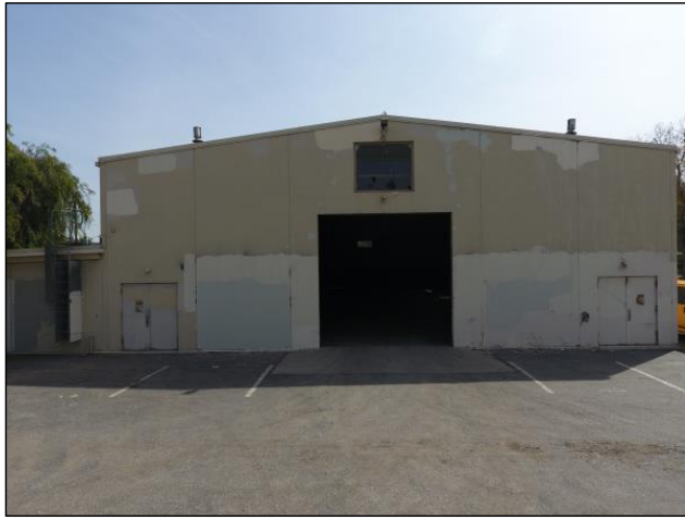
Figure 4: Northwest (rear) elevation (EOMA, 2018)
