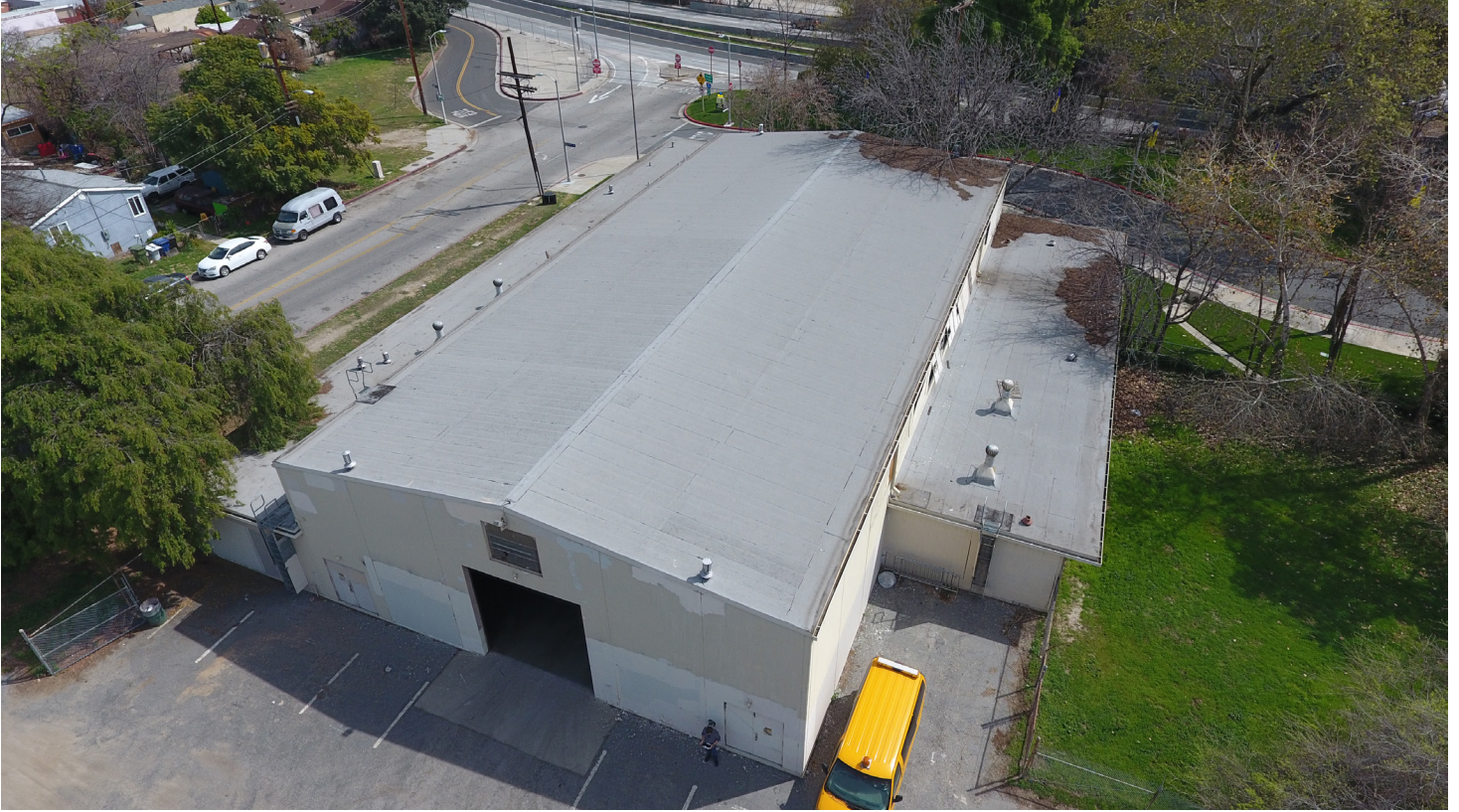
▲ Aerial view of the existing building towards 110 Freeway
