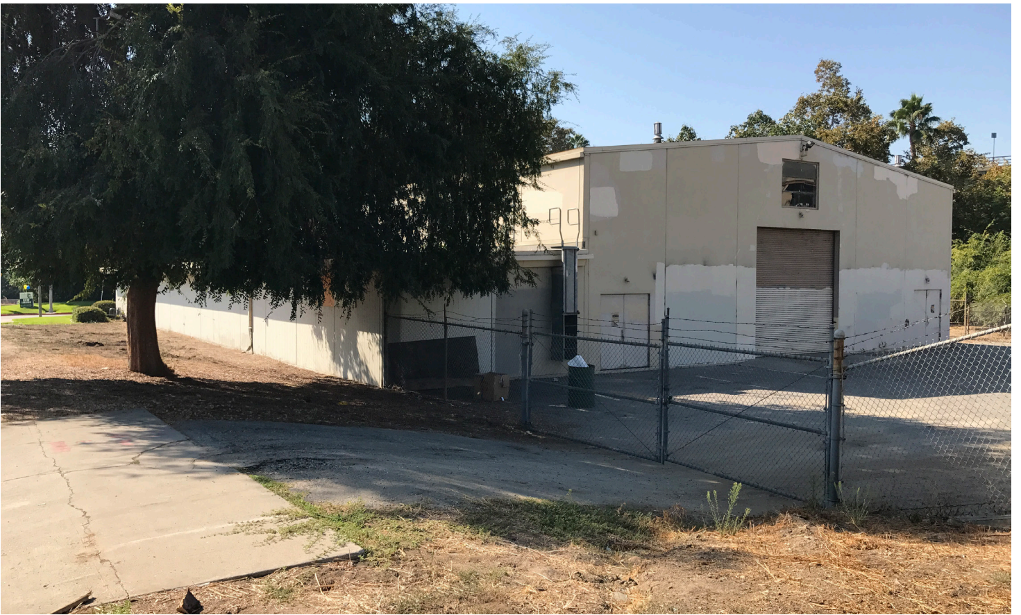
▲ West elevation, the parking lot entrance from Salonica Street
