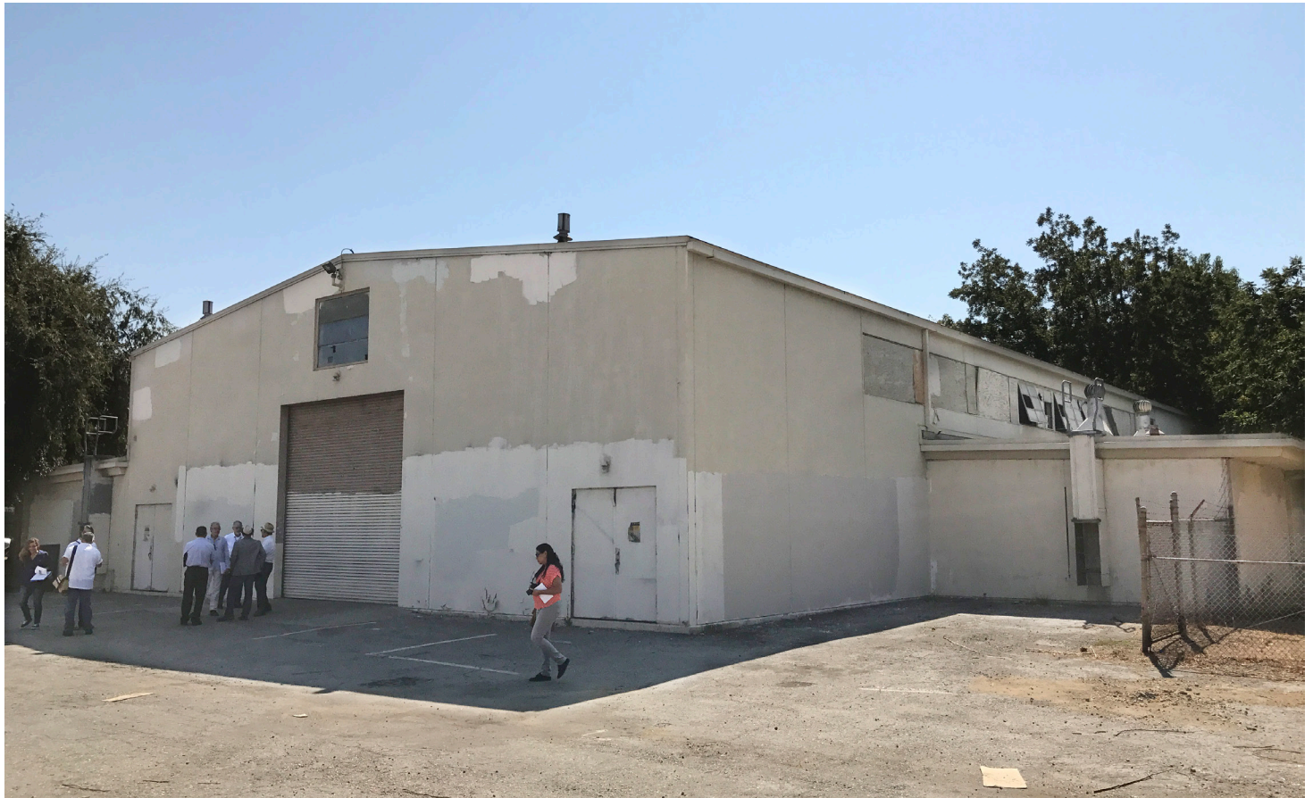
West elevation from the parking lot ▼
