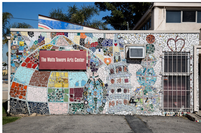
▲ Exterior - Mosaic wall reflects the work of Simon Rodia on the Watts Towers.
