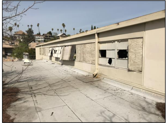
Figure 7: Clerestory windows along multipurpose space (EOMA, 2018)
