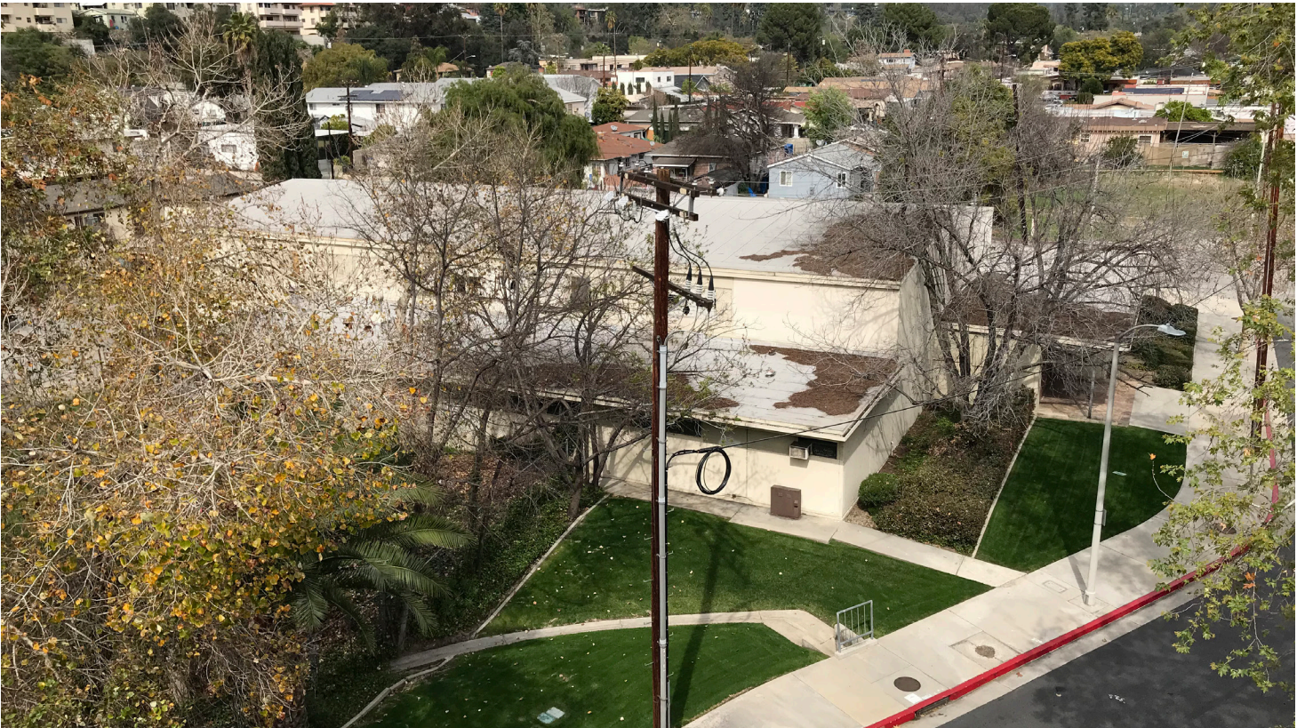
Aerial view of the existing building from York Boulevard ▼
