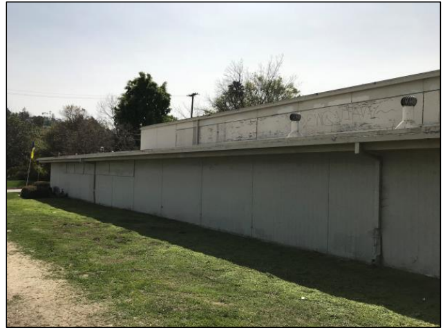
Figure 5: Northeast (side) elevation along Salonica Street (EOMA, 2018)
