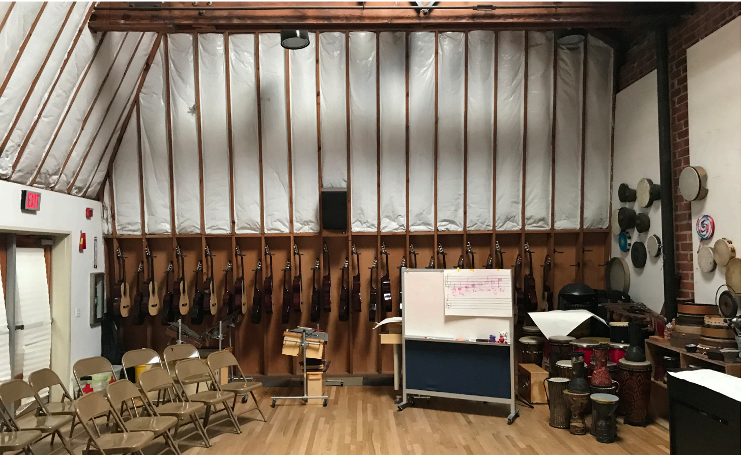
Studio - Music - Acoustic baffles and instrument storage are integrated within the exposed structure of the walls. ▼
