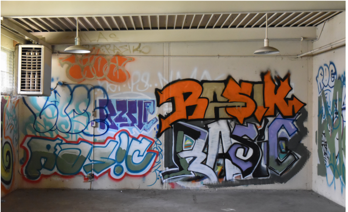
Interior of the perimeter single-height space ▼
