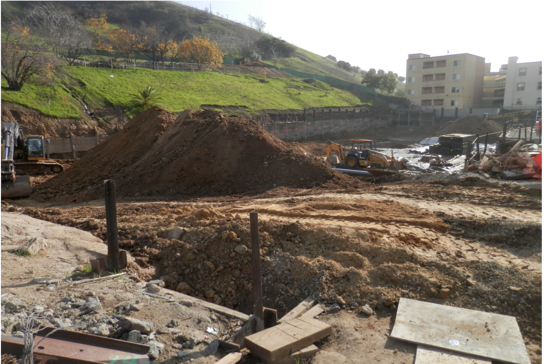
View from inside the construction fence at 4208 E. Huntington Dr. South.
