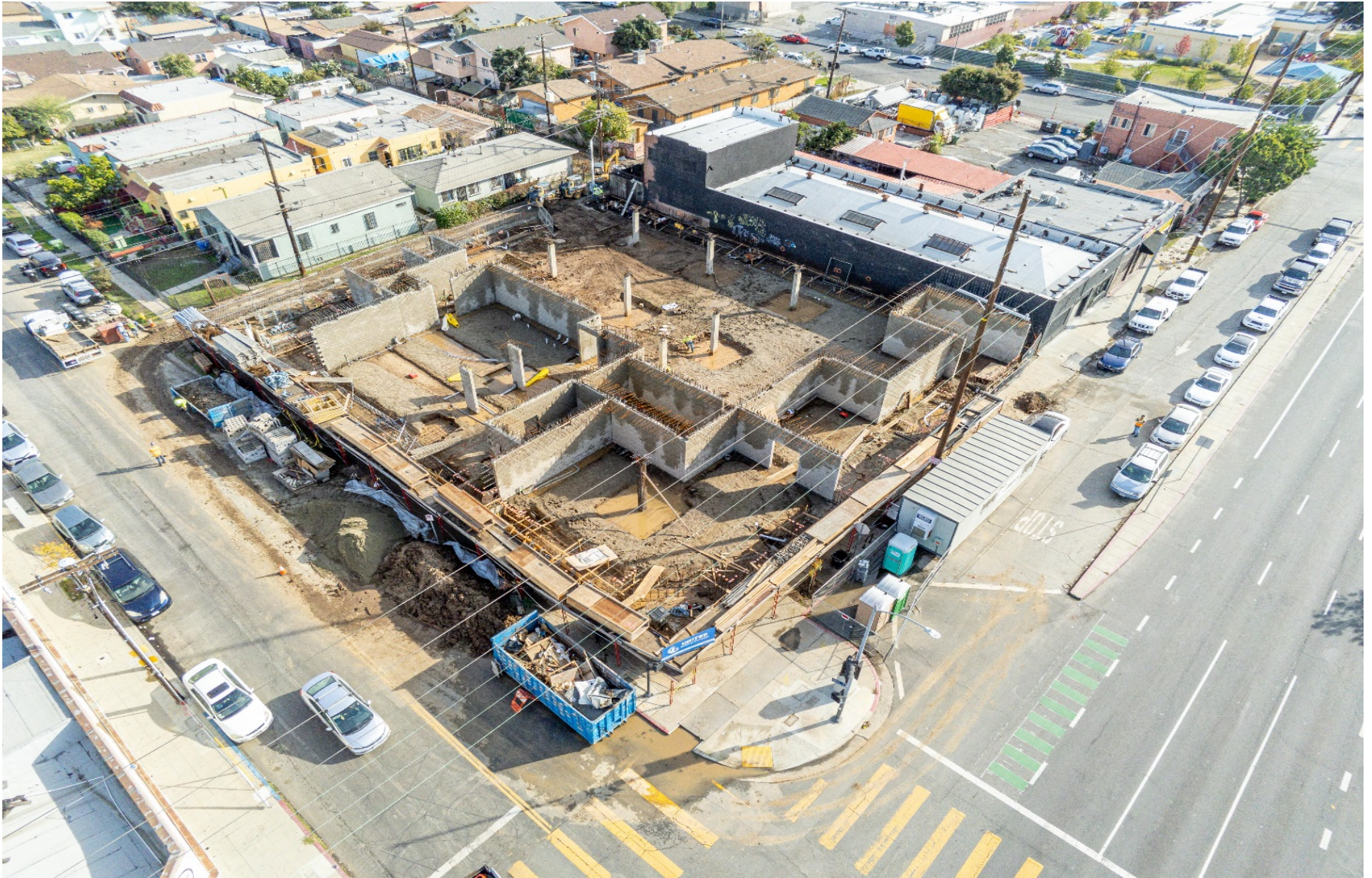
View from overhead of the construction site at 7600 S Vermont.
