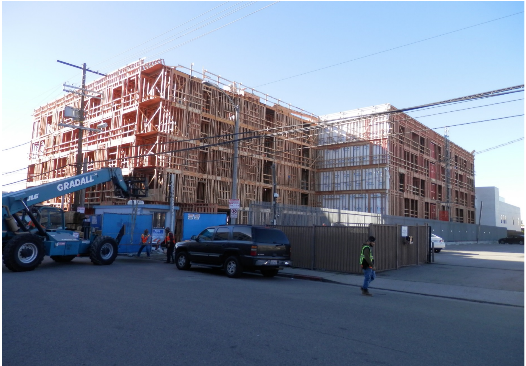
Located at 1119 N. Mc Cadden Pl. Street view from front of site on Las Palmas St.
