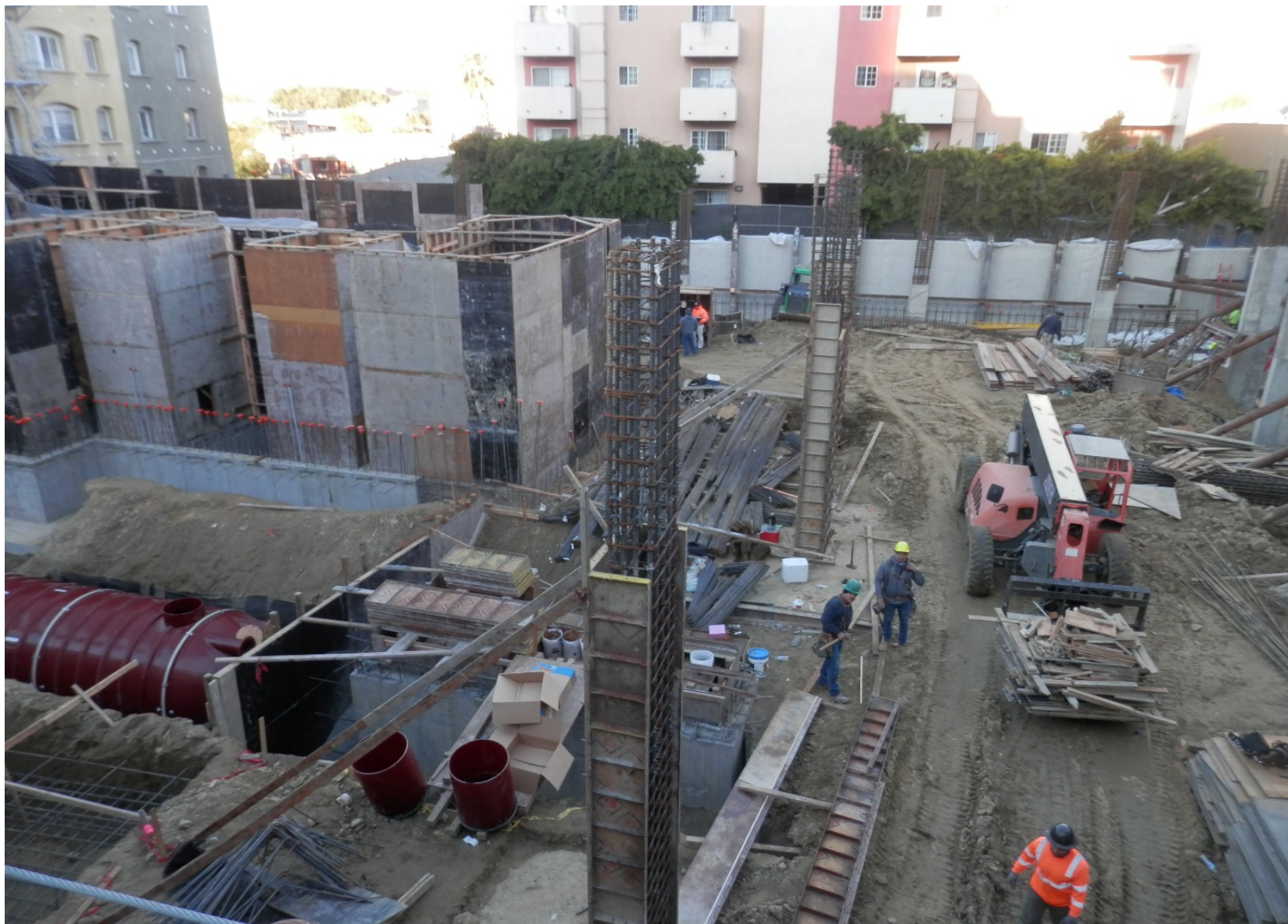
View from inside the construction fence at 445 S. Harford Ave.
