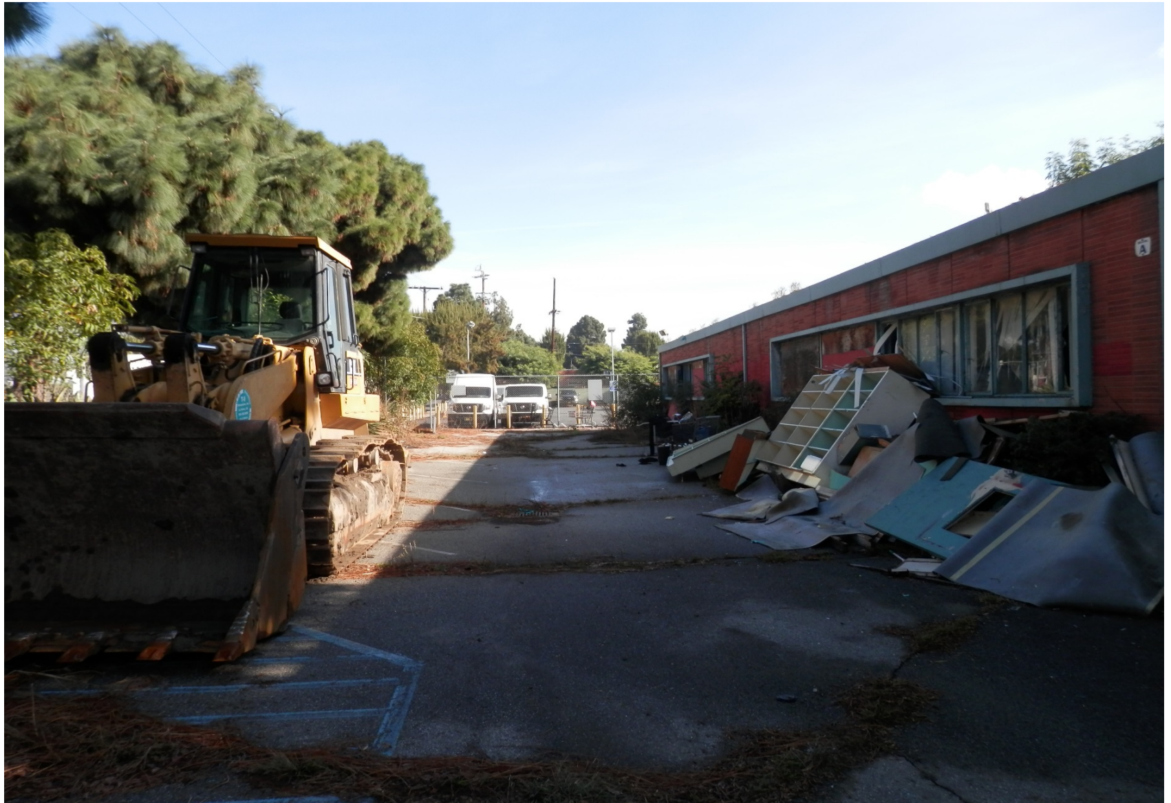
View from just inside the construction fence at 11950 W. Missouri St.
