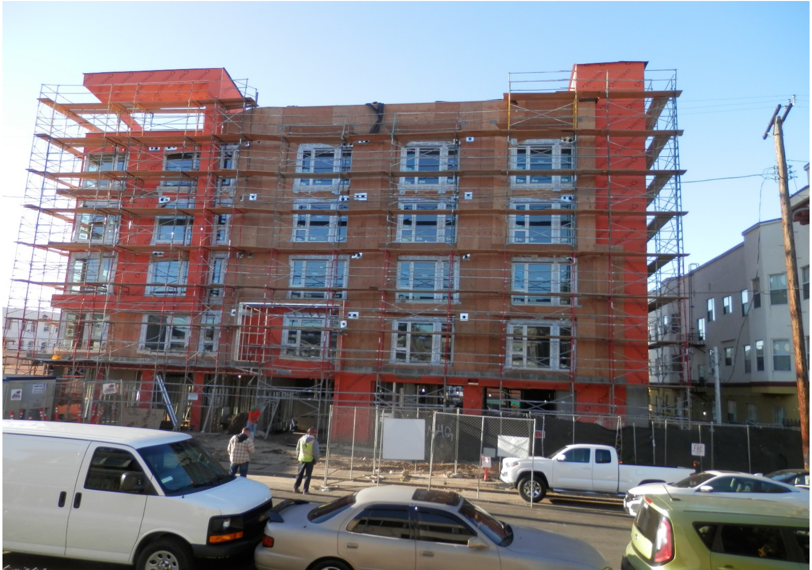
Located at 1532-38 Cambria St. View from across the street of site.
