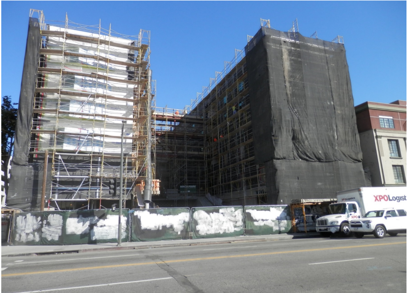
Located at 401 E 7 th St. View from across the street.
