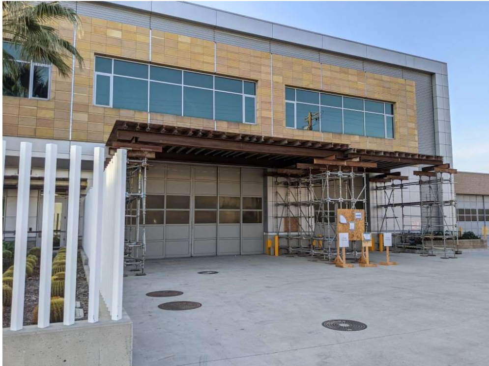
North side of facility. Erected scaffolding over FS4 firetruck entrances
