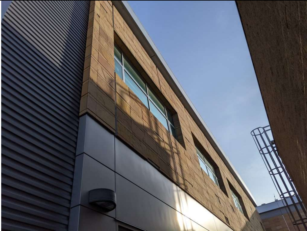
South-facing side of EOC facility
