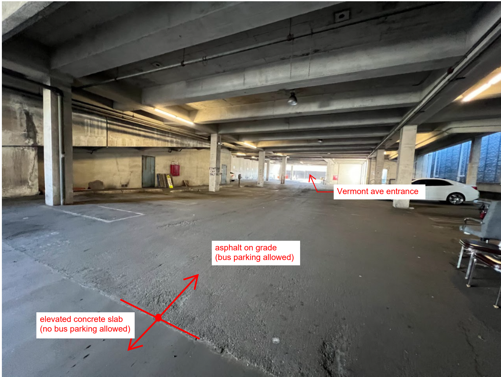
PHOTO-3: 1 ST FLOOR FROM VERMONT AVE ENTRANCE
