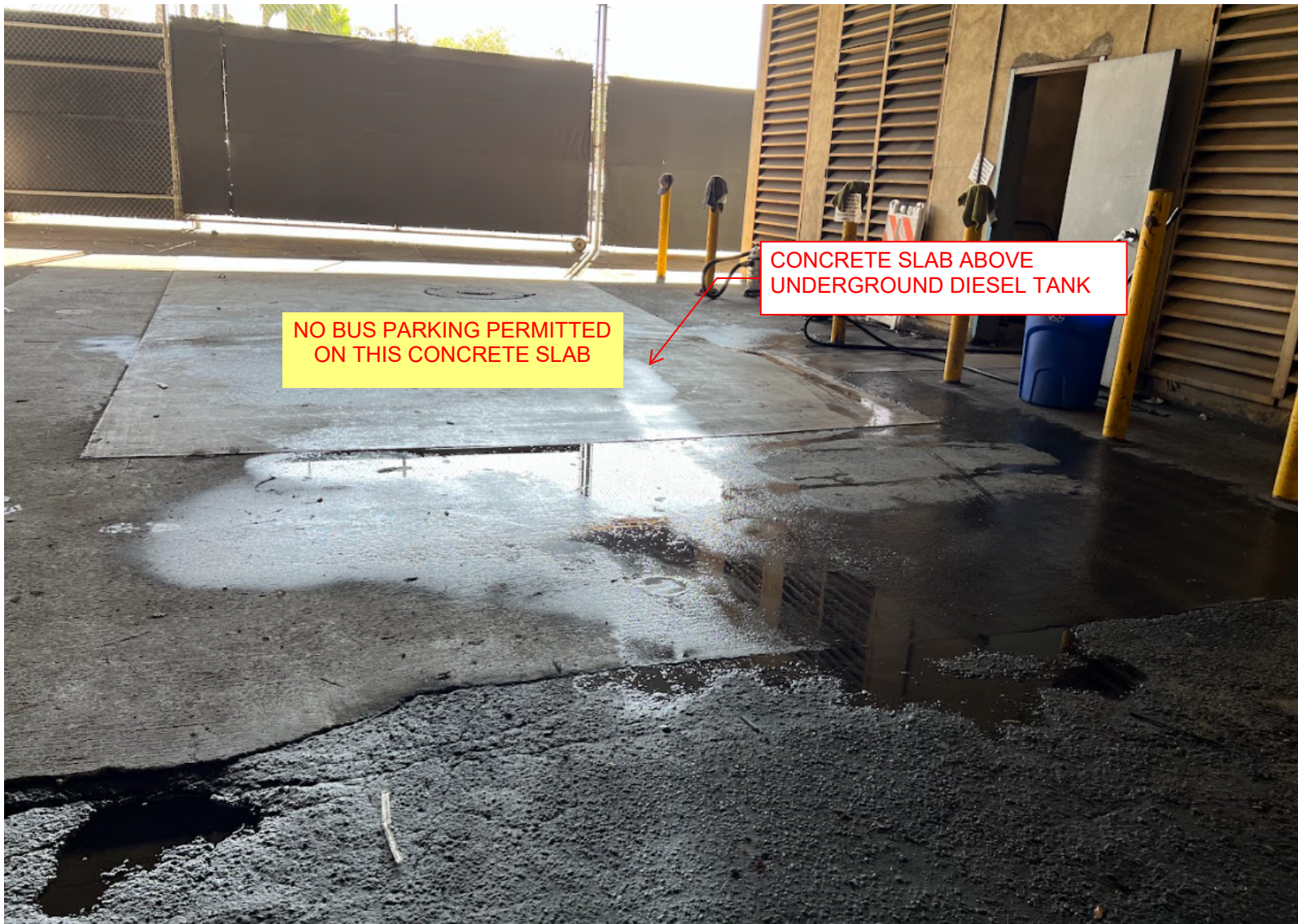
PHOTO-2: VERMONT AVE ENTRANCE
