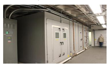
Picture 04: Installed Chiller Plant & Completed Mechanical Room on P3
