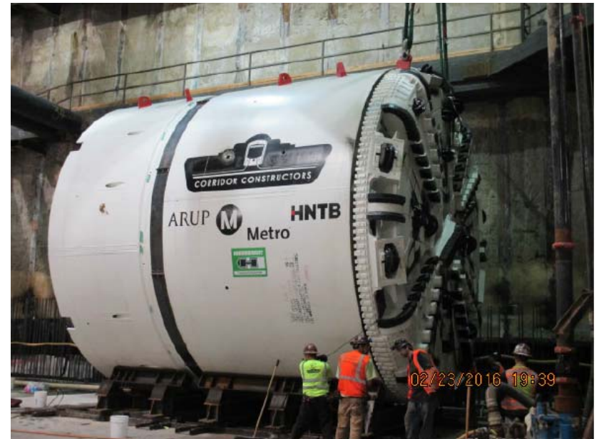
Exposition/Crenshaw Station – Tunnel Boring Machine – “Harriet”
