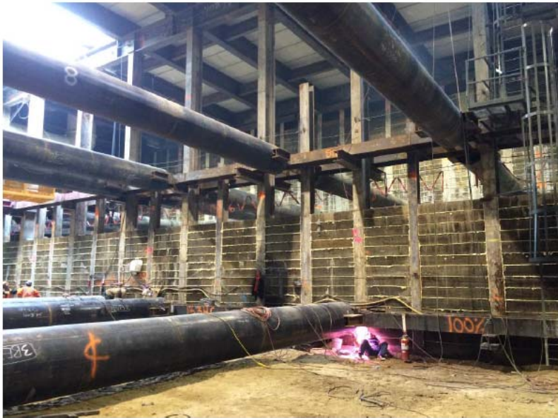
Leimert Park Station – Tier 2 strut installation
