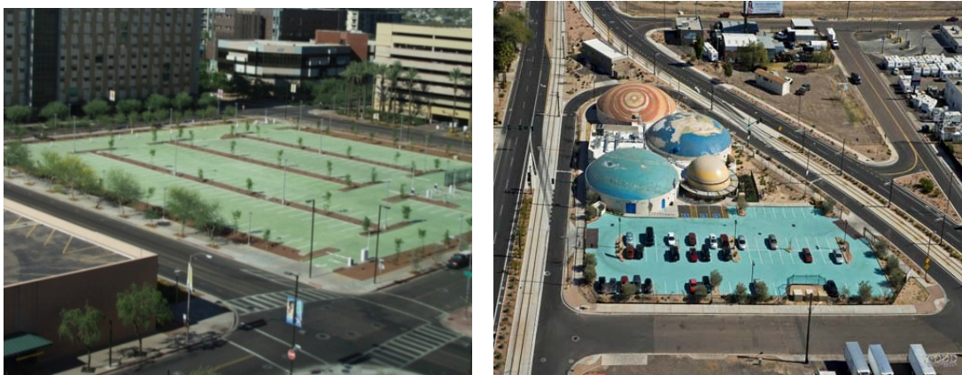
FIGURE 17. SHERATON HOTEL (LEFT) AND DUFFY CHARTER SCHOOL (RIGHT), BOTH IN PHOENIX, AZ (EMERALD CITIES).
