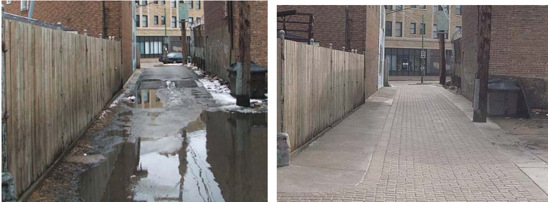
FIGURE 18. ALLEY WITH IMPERMEABLE PAVEMENT AND POOR DRAINAGE (LEFT) AND ALLEY INCORPORATING GREEN ALLEY PRINCIPLES (RIGHT) (CDOT).
