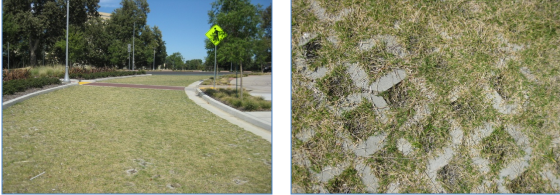
FIGURE 13. VEGETATED CONCRETE GRID PAVERS
