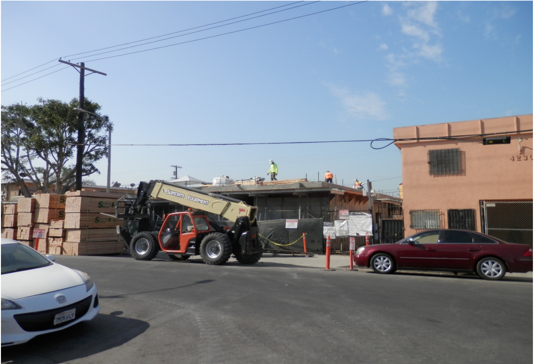
View from across the street at 4220 Montclair St.
