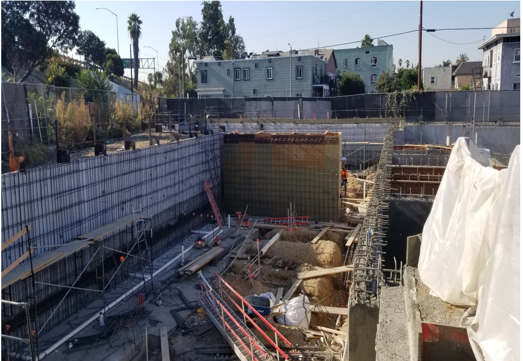
View from inside the fence at 720 W. Washington Blvd.
