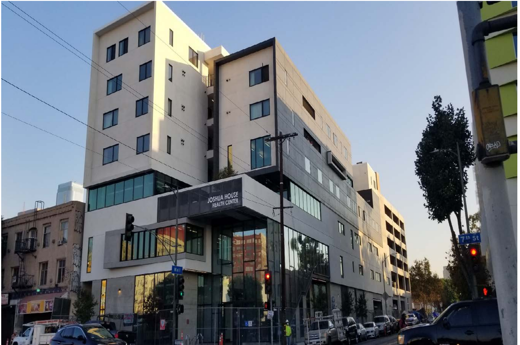
Located at 649 S. Wall St. View from across the street of 7 th St. & Wall St.
