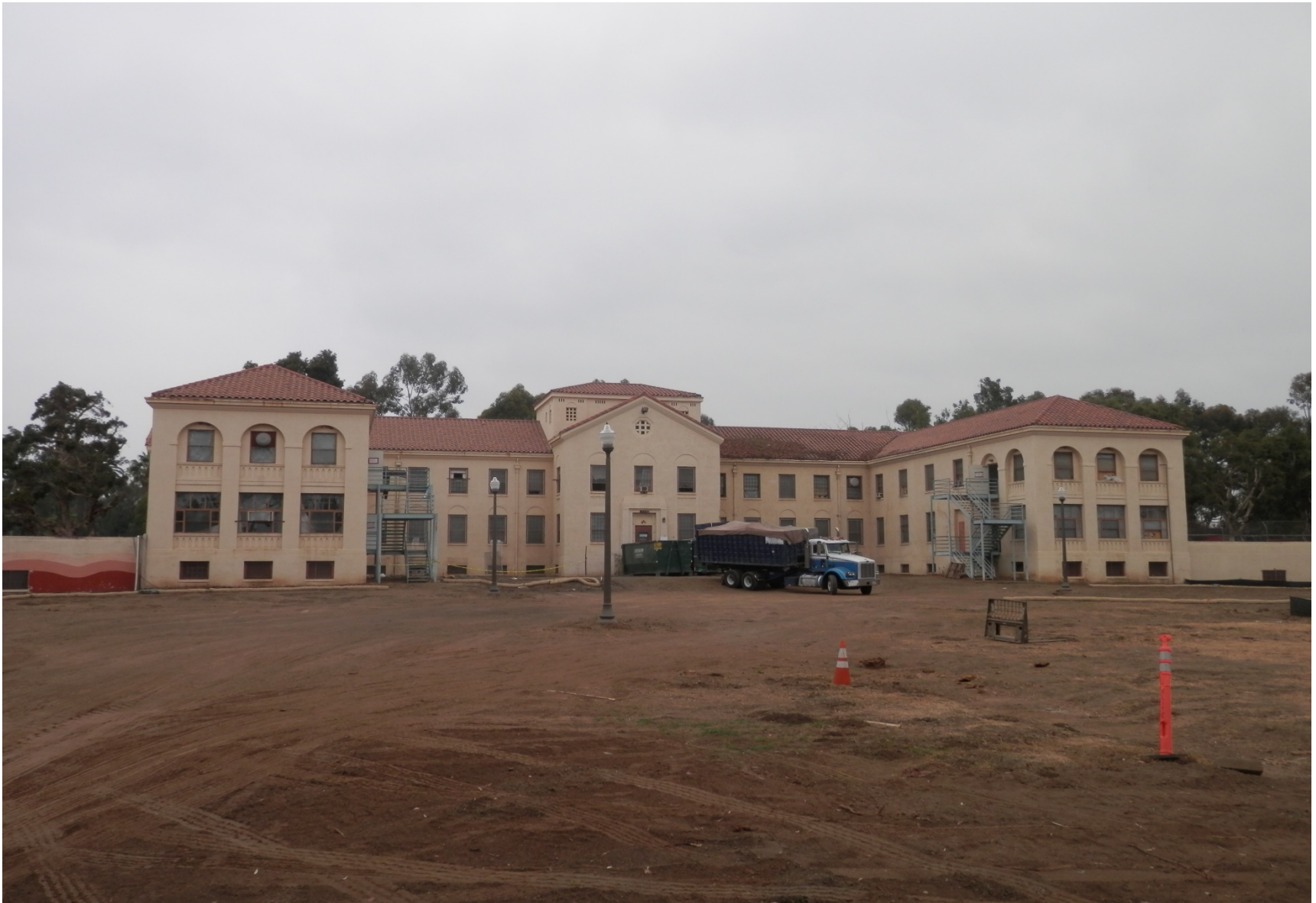
View from the Building 205 and Building 208 courtyard at 11301 Wilshire Blvd.
