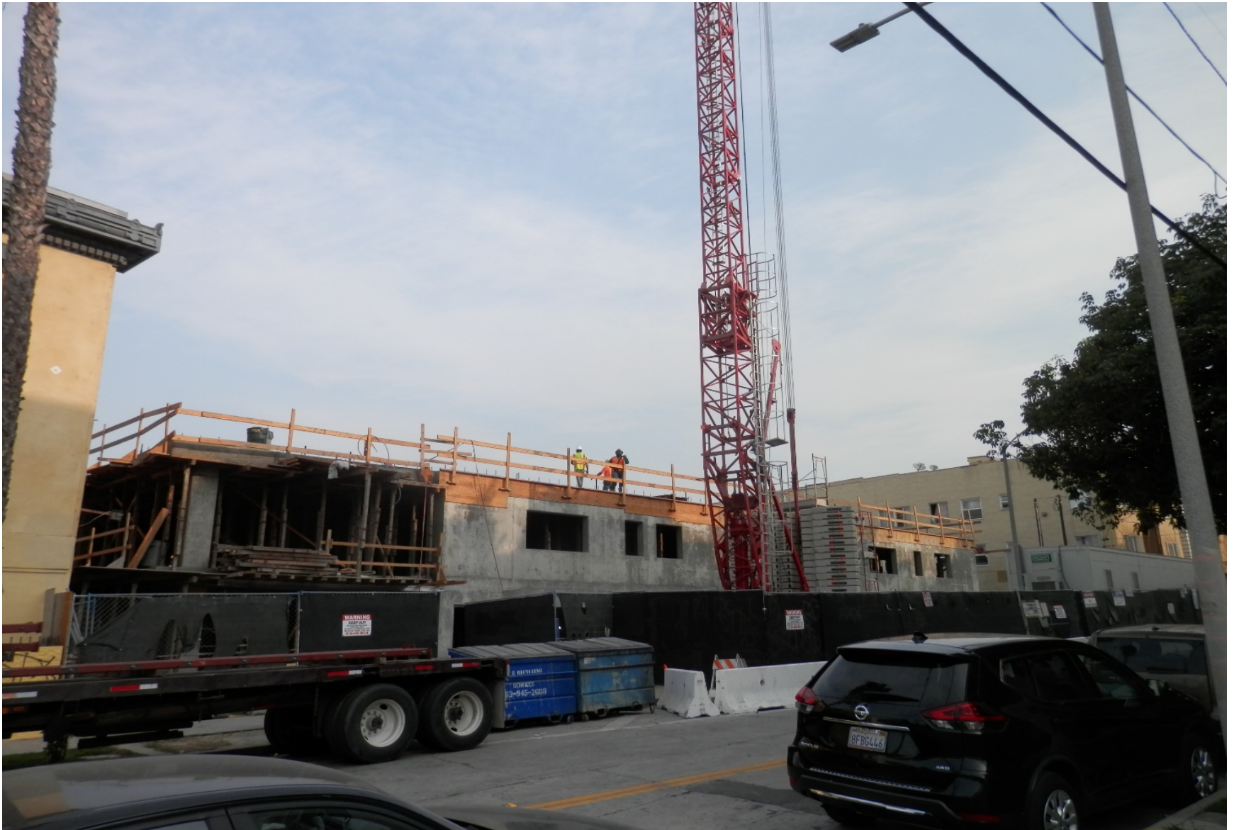
View from across the street at 445 S. Harford Ave.
