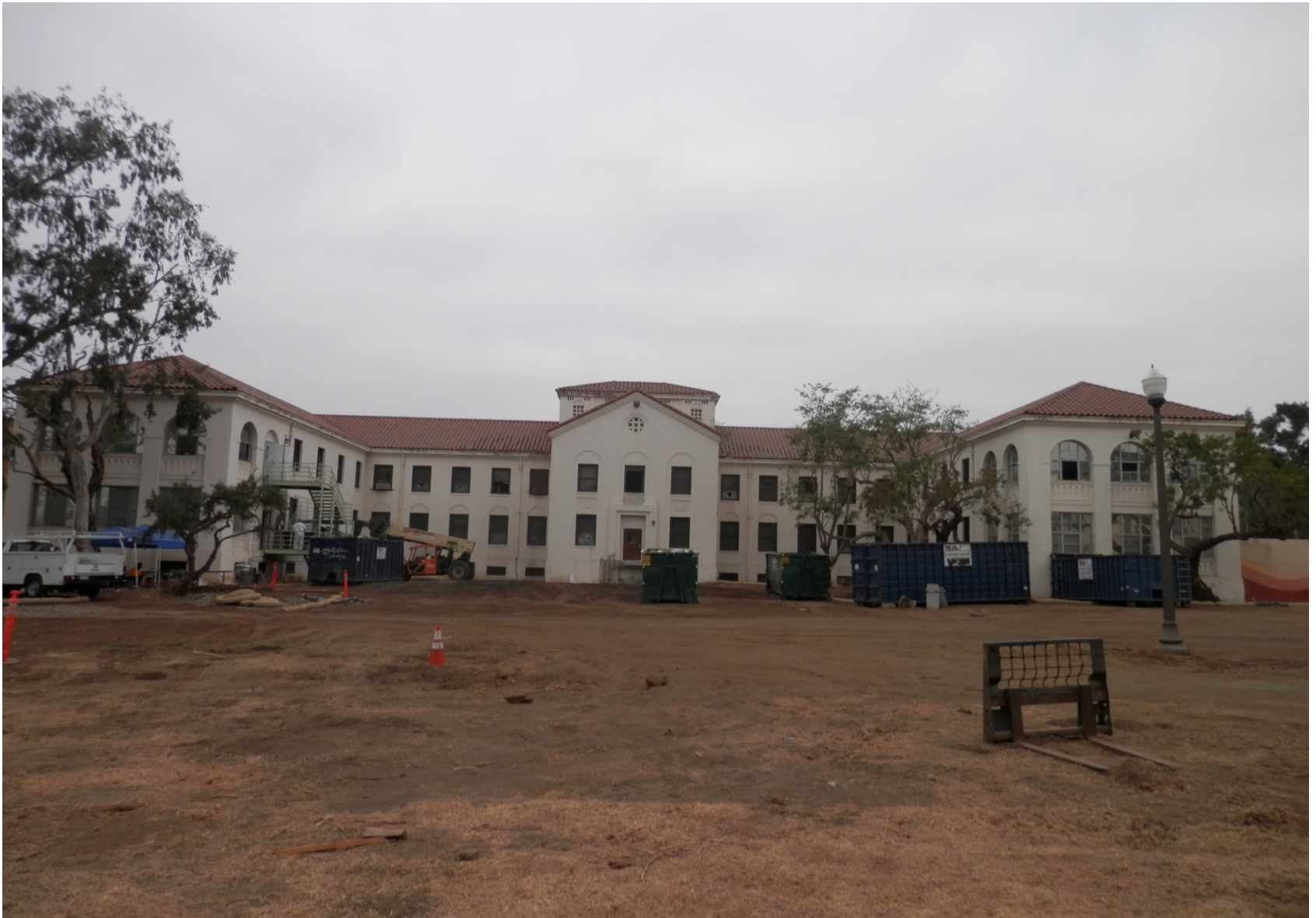
View from the Building 205 and Building 208 courtyard at 11301 Wilshire Blvd.
