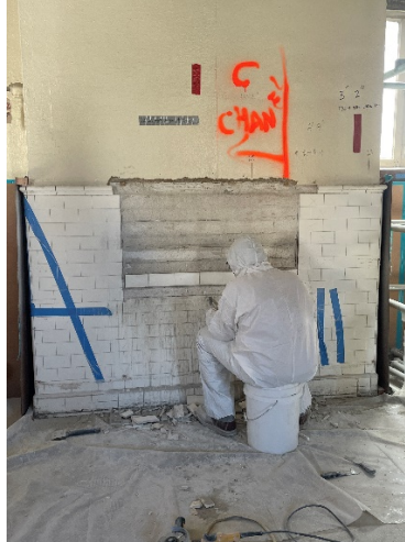
Historic Tile Preservation
