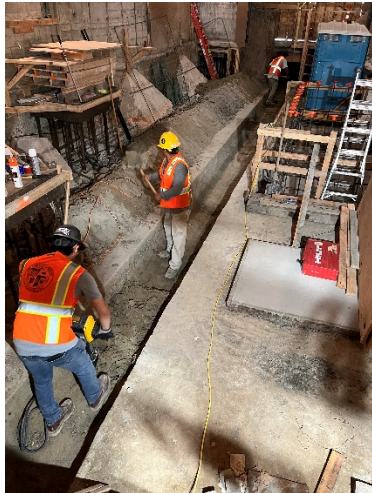
Pyramidal Foundations Repair
