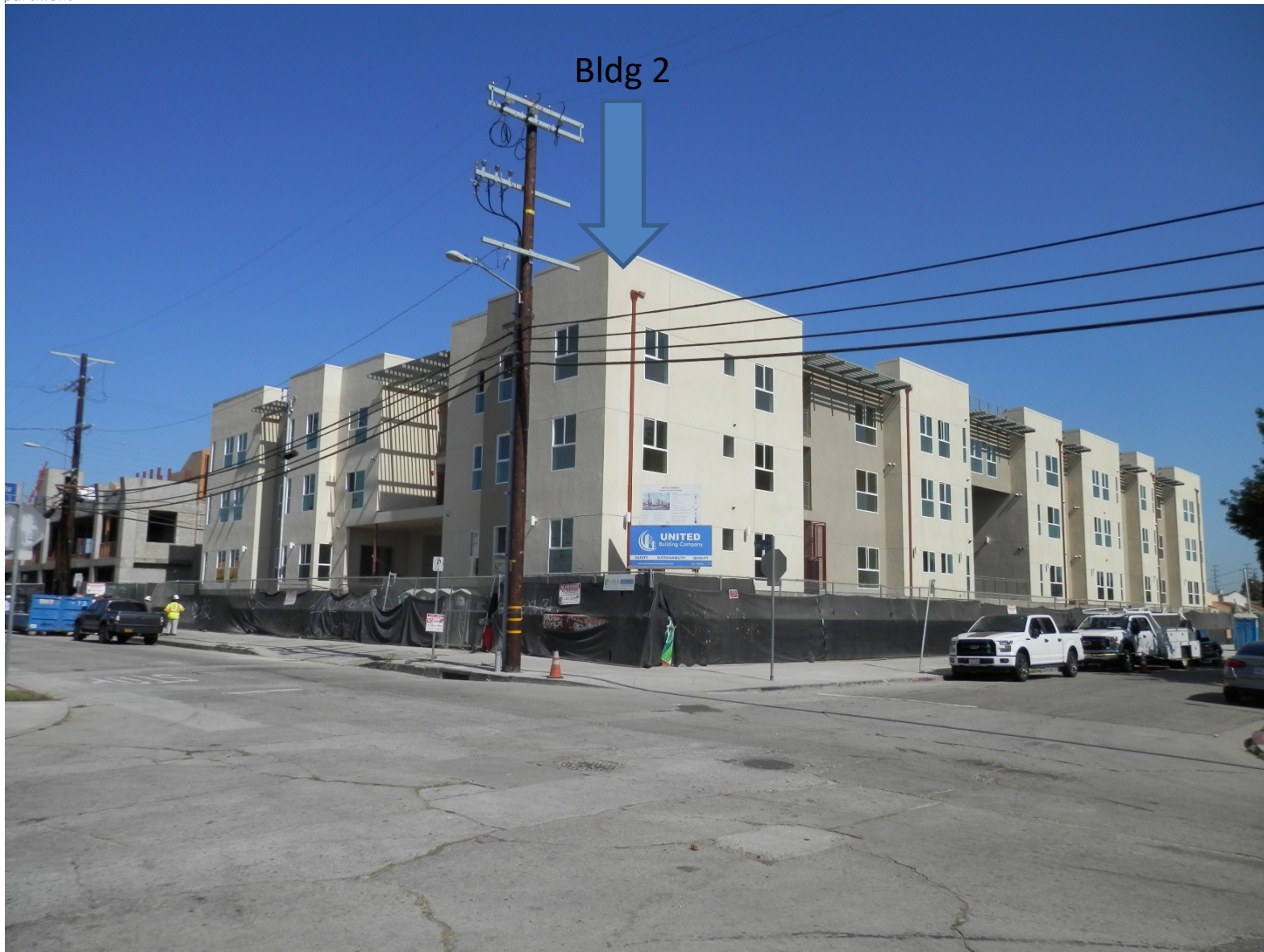
Located at 8707-27 S. Menlo Apts. Bldg 2 residential. View from Menlo & 88 th .
