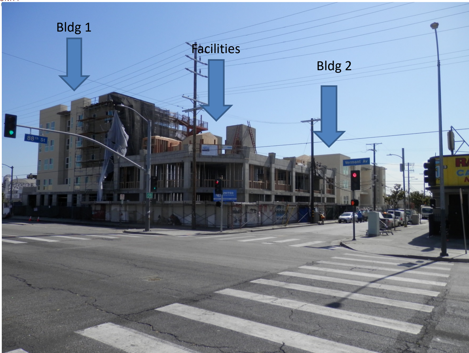
Located at 8707-27 S. Vermont. Building 1 & facilities view from 88th & Vermont.
