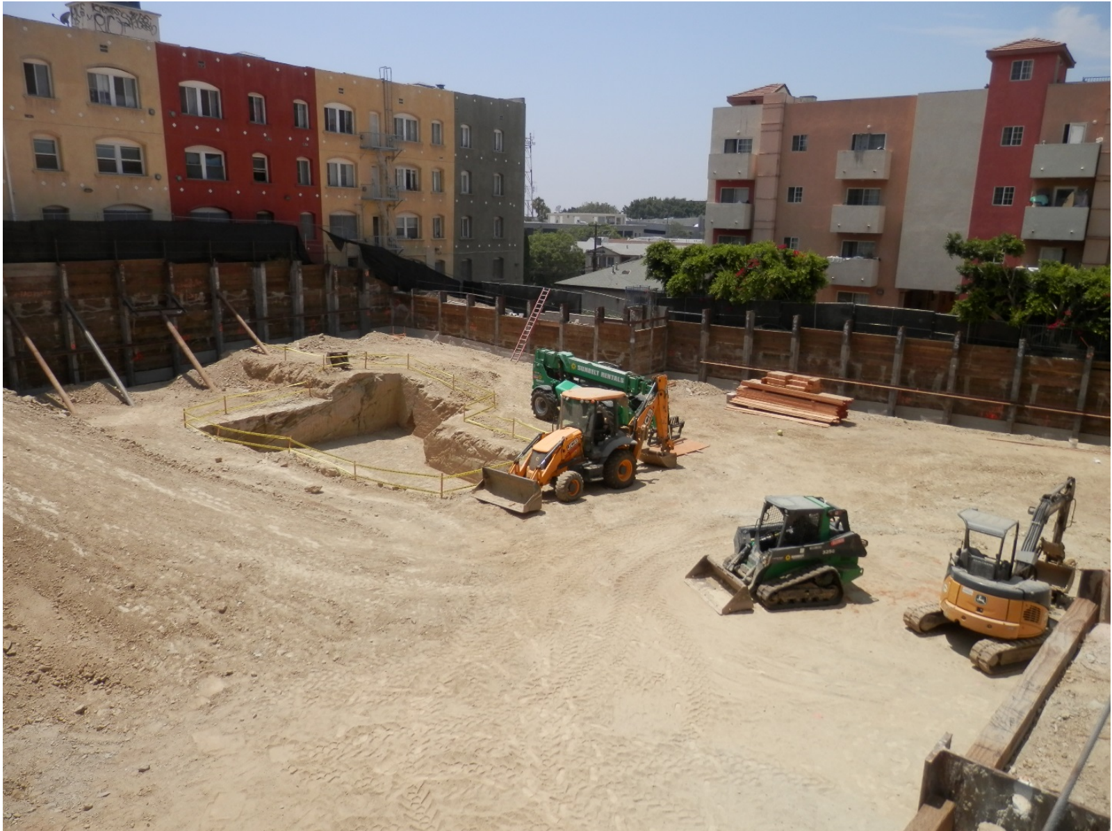
View from just inside fence at 445 S. Harford Ave.
