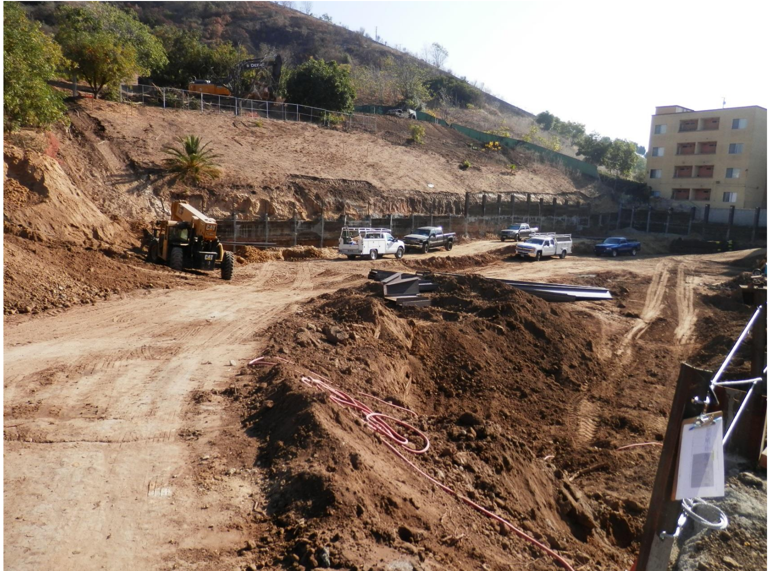
View from inside the construction fence at 4208 E. Huntington Dr. South.
