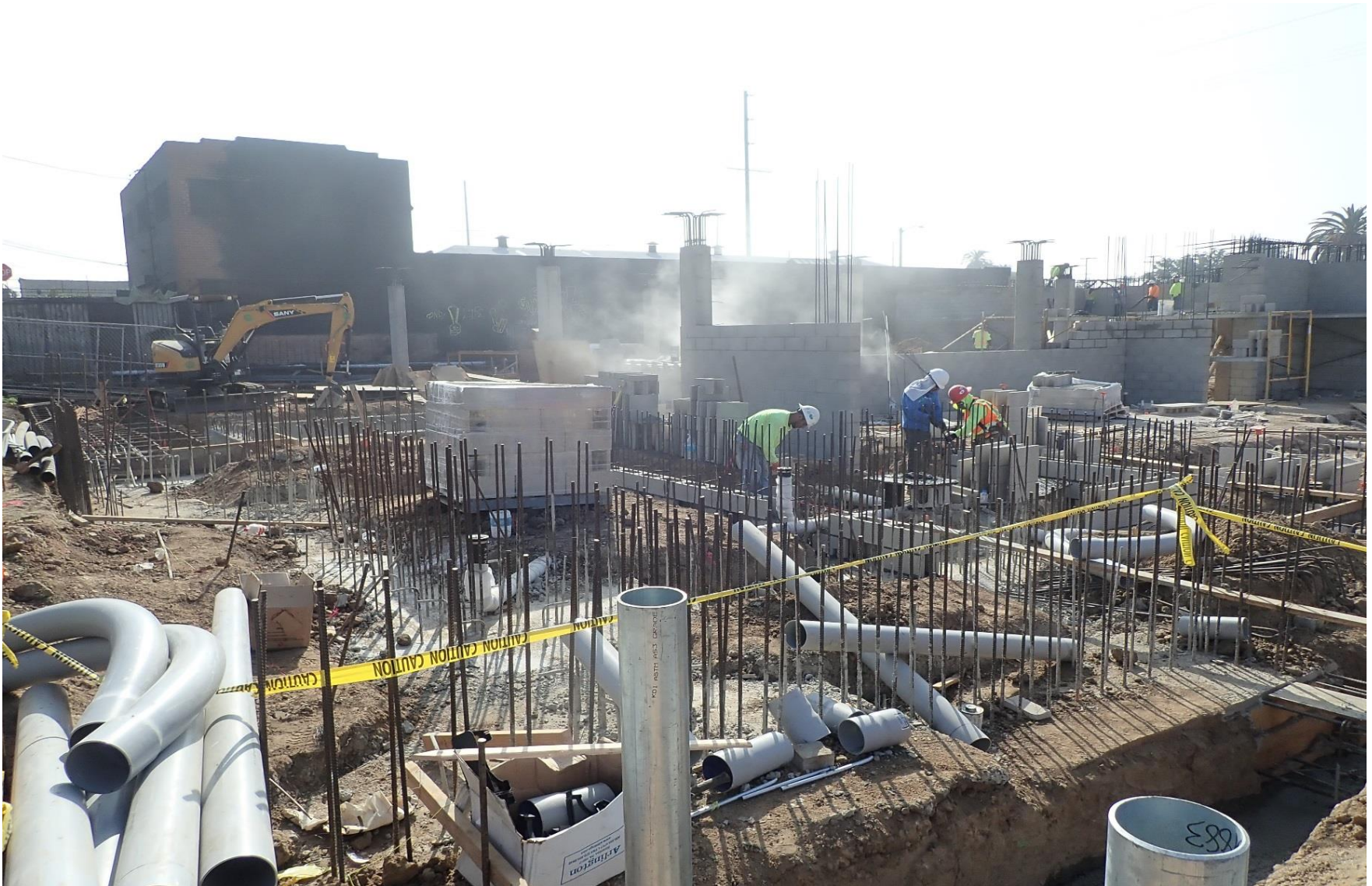
View from inside of the construction fence at 7600 S Vermont.
