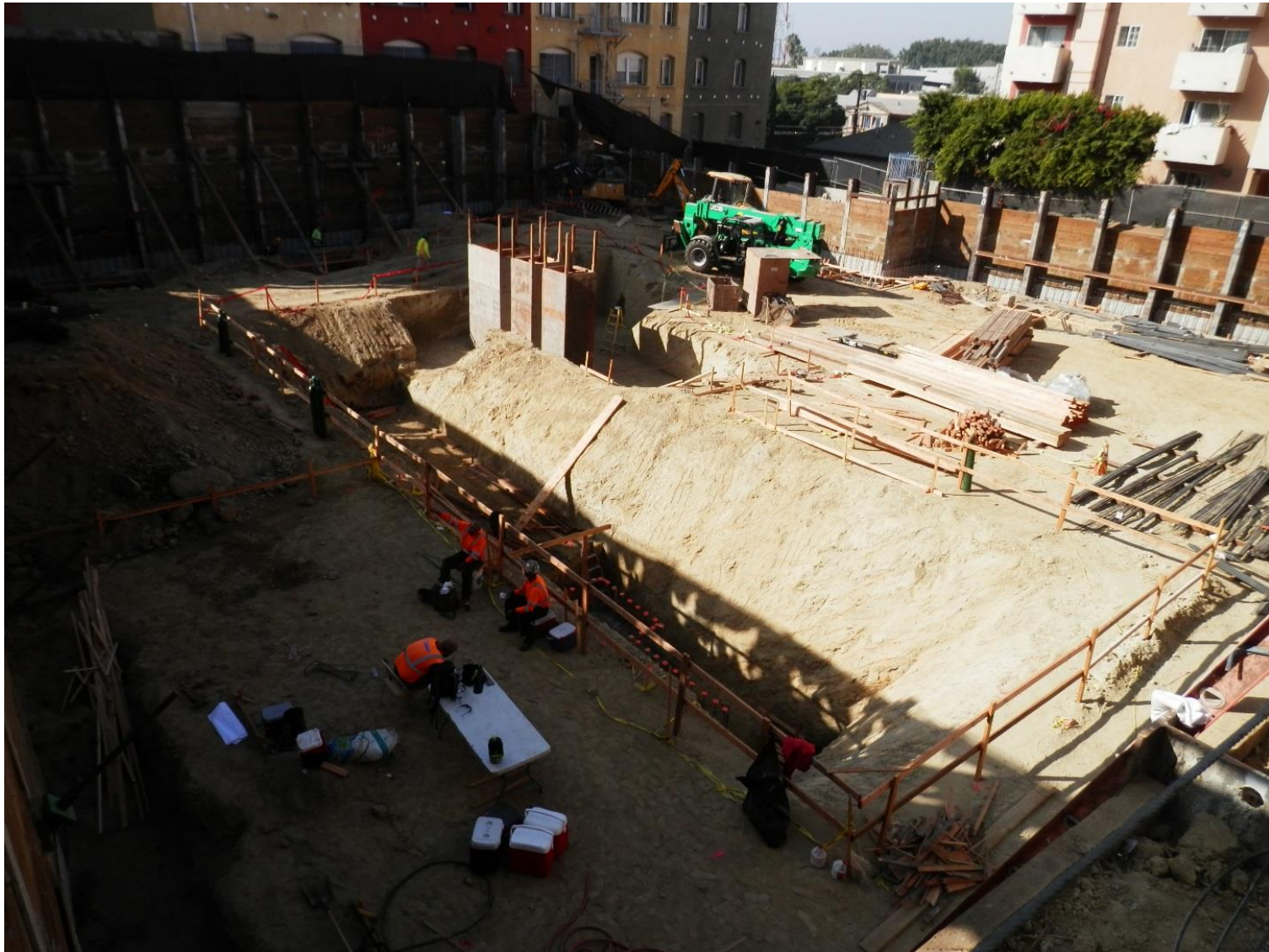
View from inside the construction fence at 445 S. Harford Ave.
