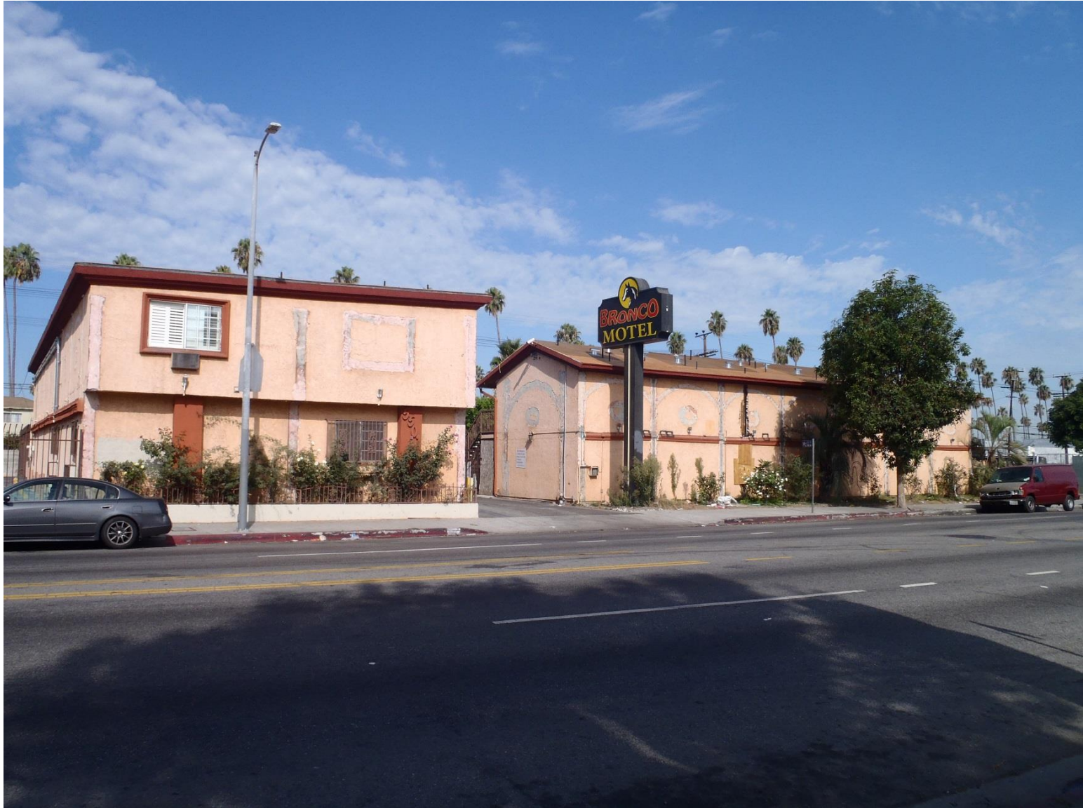
View from across site at 5501 S. Western Ave.
