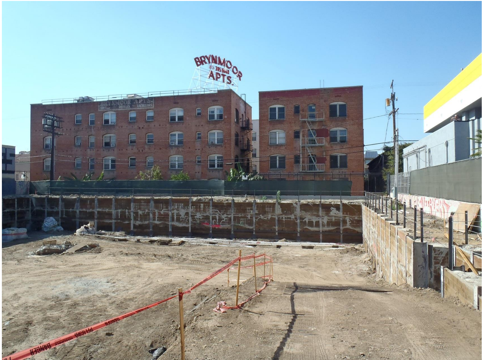
View from inside of the construction fence at 433 S Vermont .
