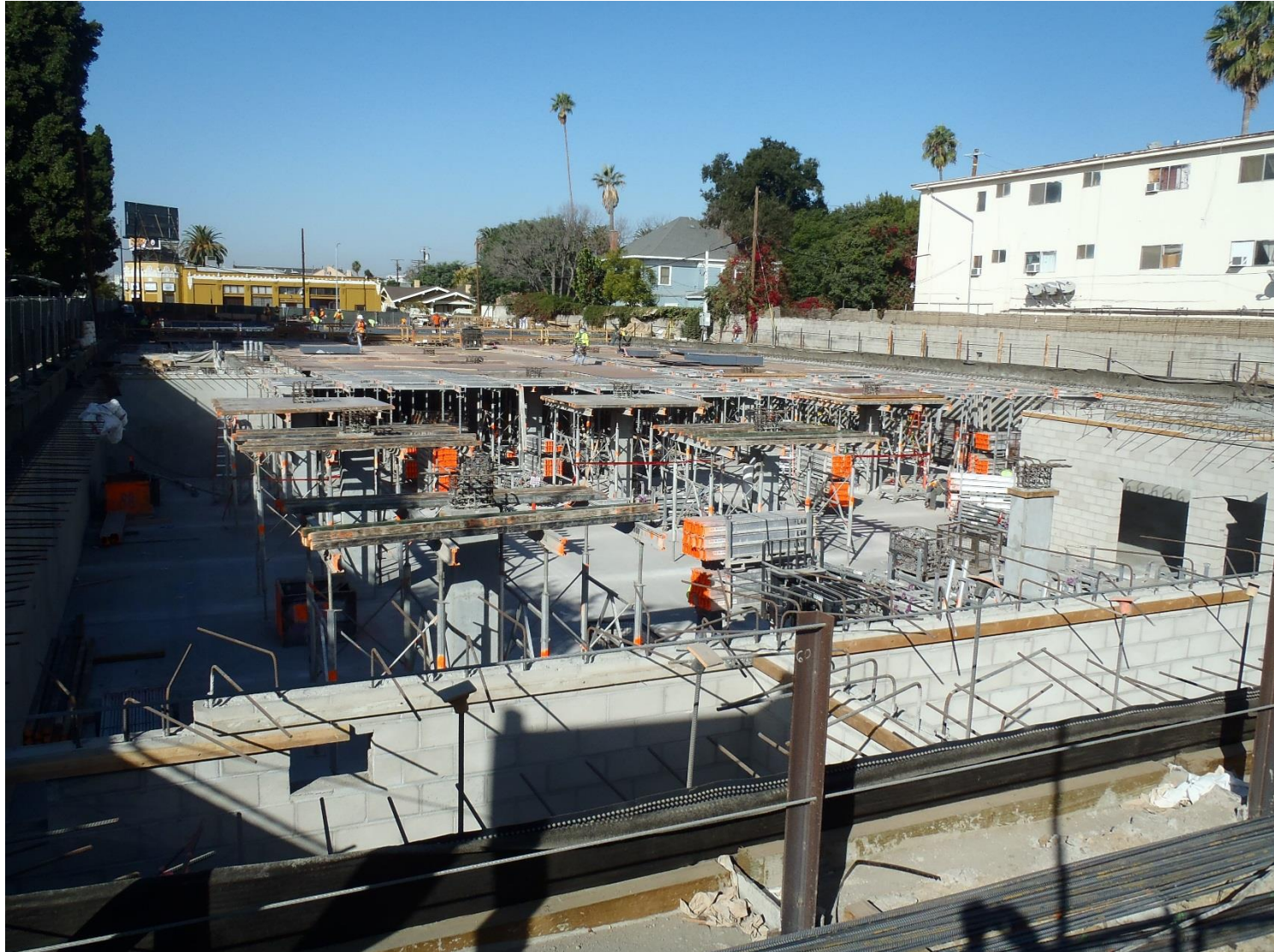
Street view from entrance to site at Washington & Gramercy. .
