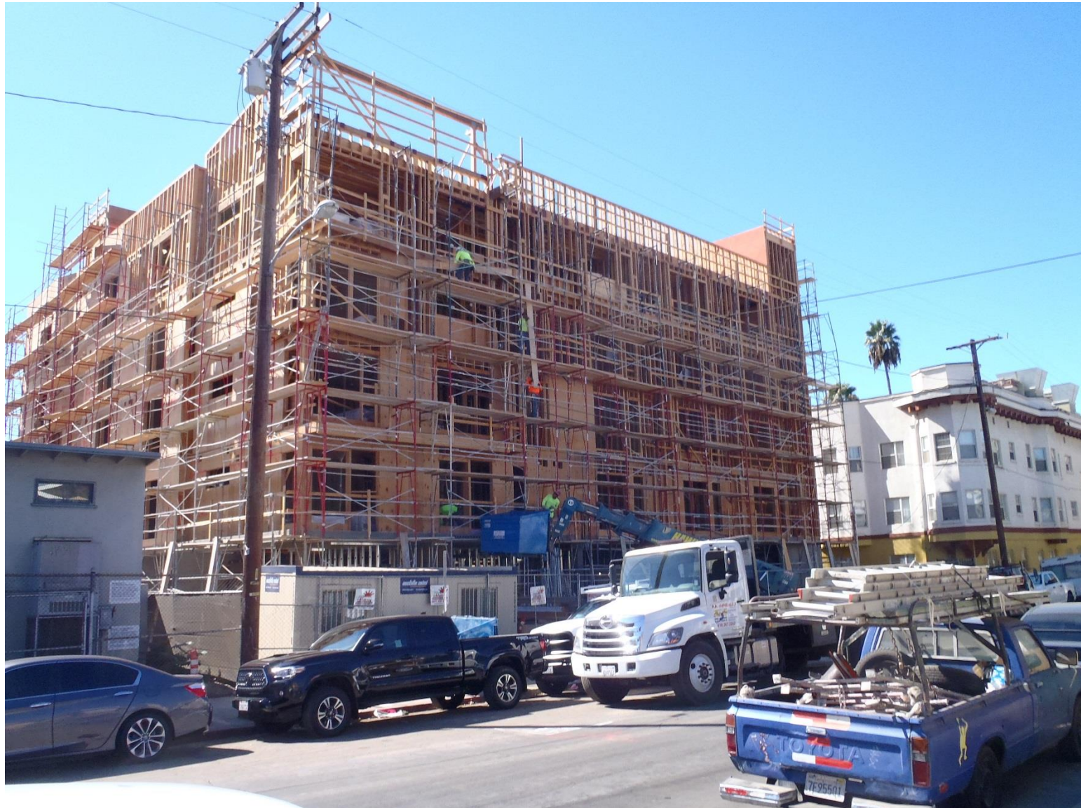
Located at 1532-38 Cambria St. View from across the street of site.
