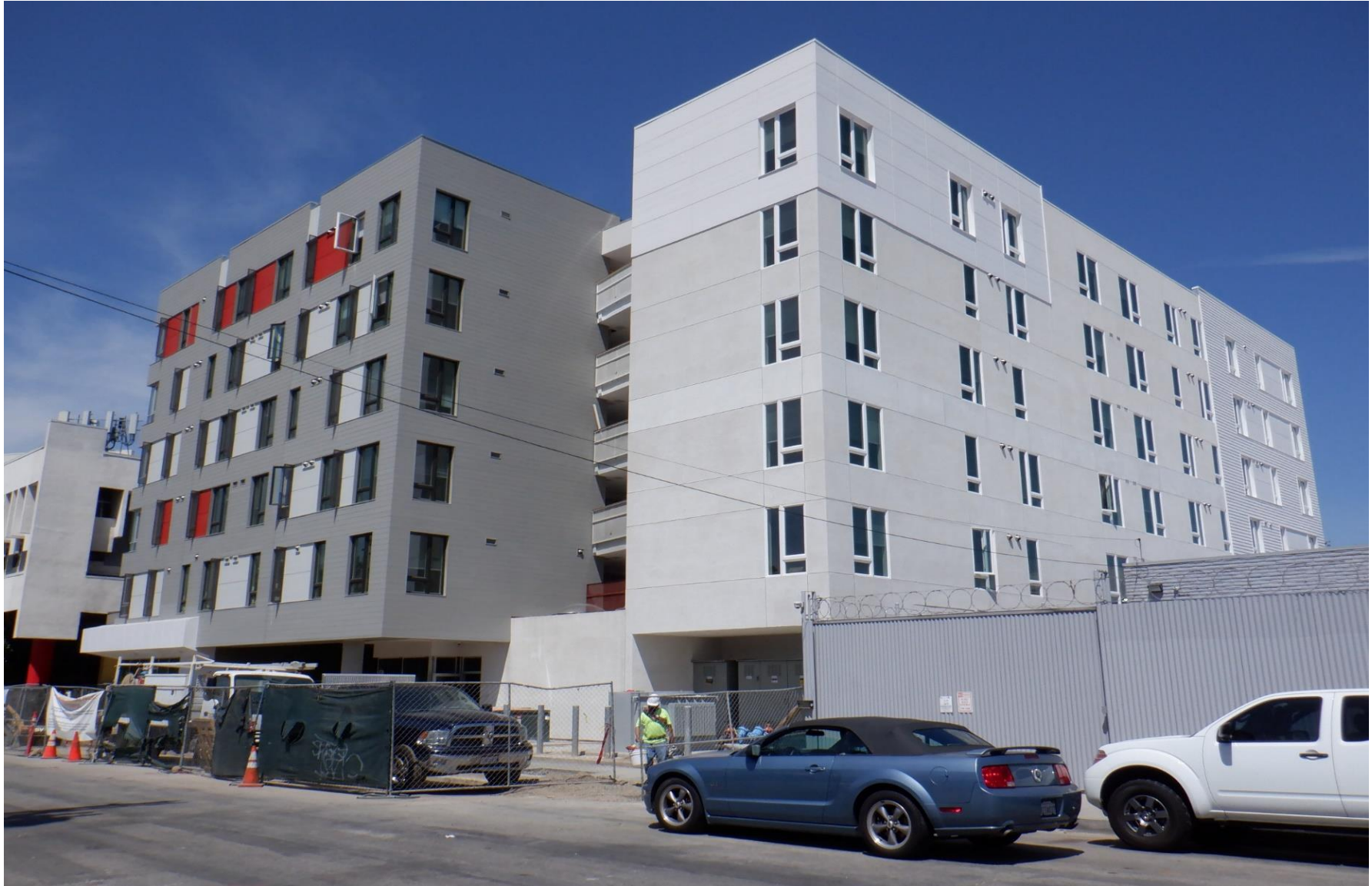
Path Metro Phase 2. View of site at corner of Beverly Blvd & Madison Ave.
