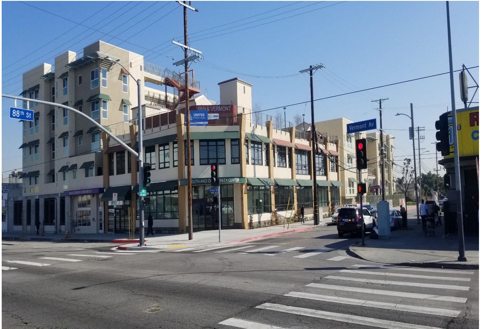
Located at 8707-27 S. Vermont. Building 2 & facilities view from 88th & Vermont.
