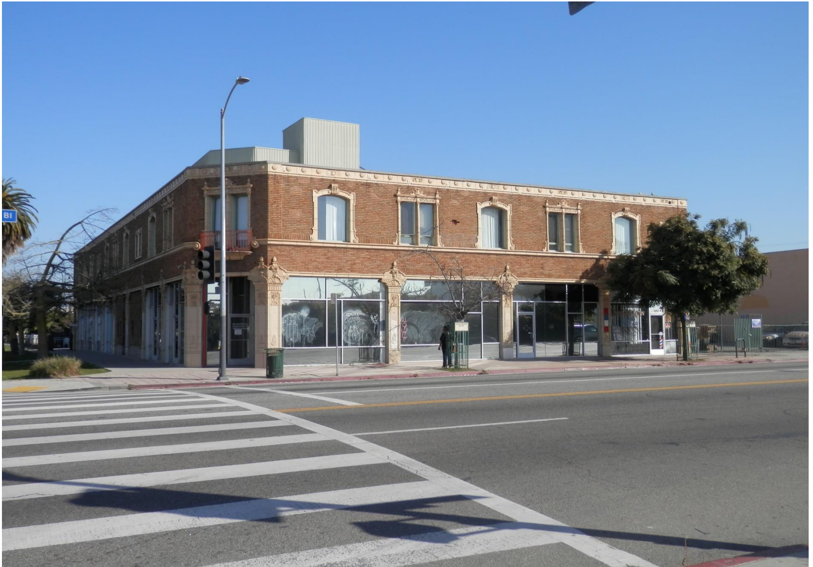
View from across the street at 4220 Montclair St.
