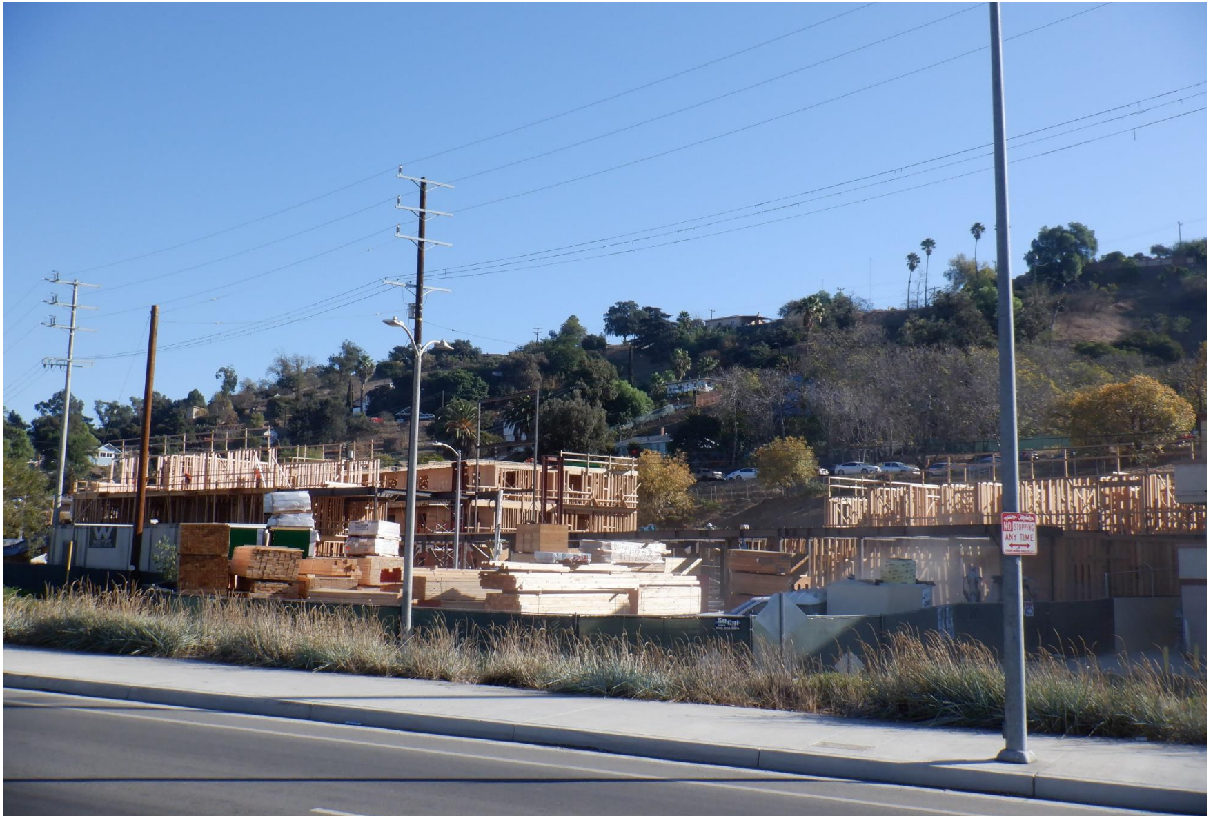
View from just inside the fence of the site at 4208 E Huntington Dr. South.
