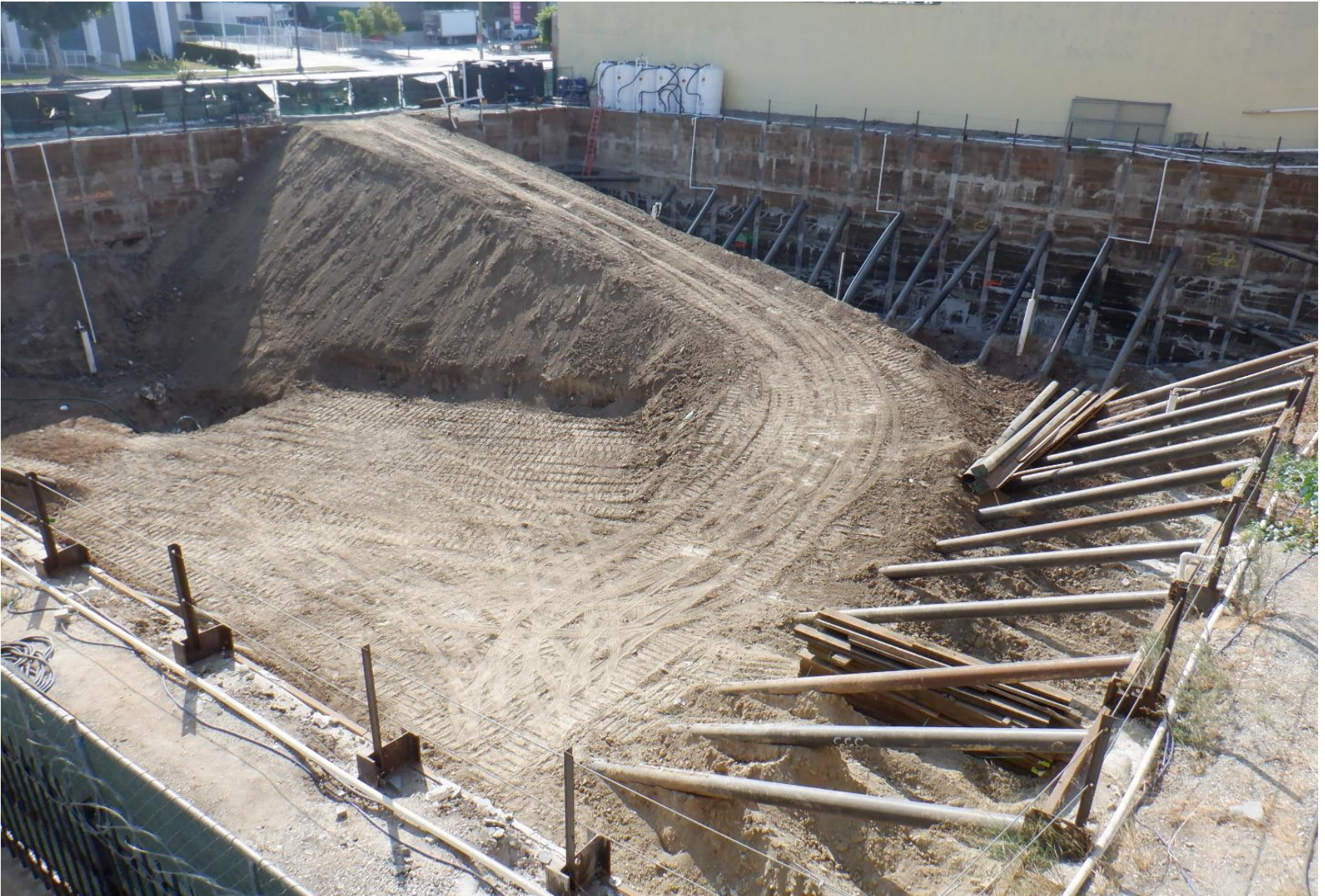
View from inside of the construction fence at 433 S Vermont.
