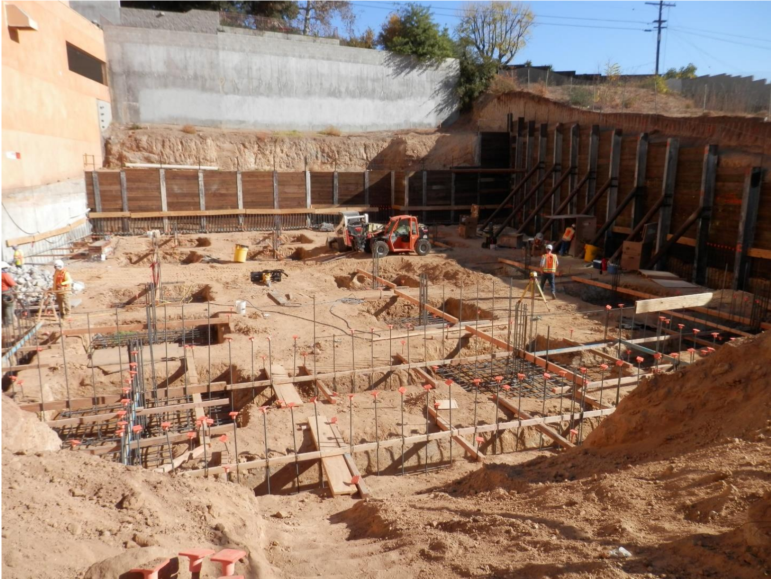
View from inside the fence at 1332 Colorado Blvd.
