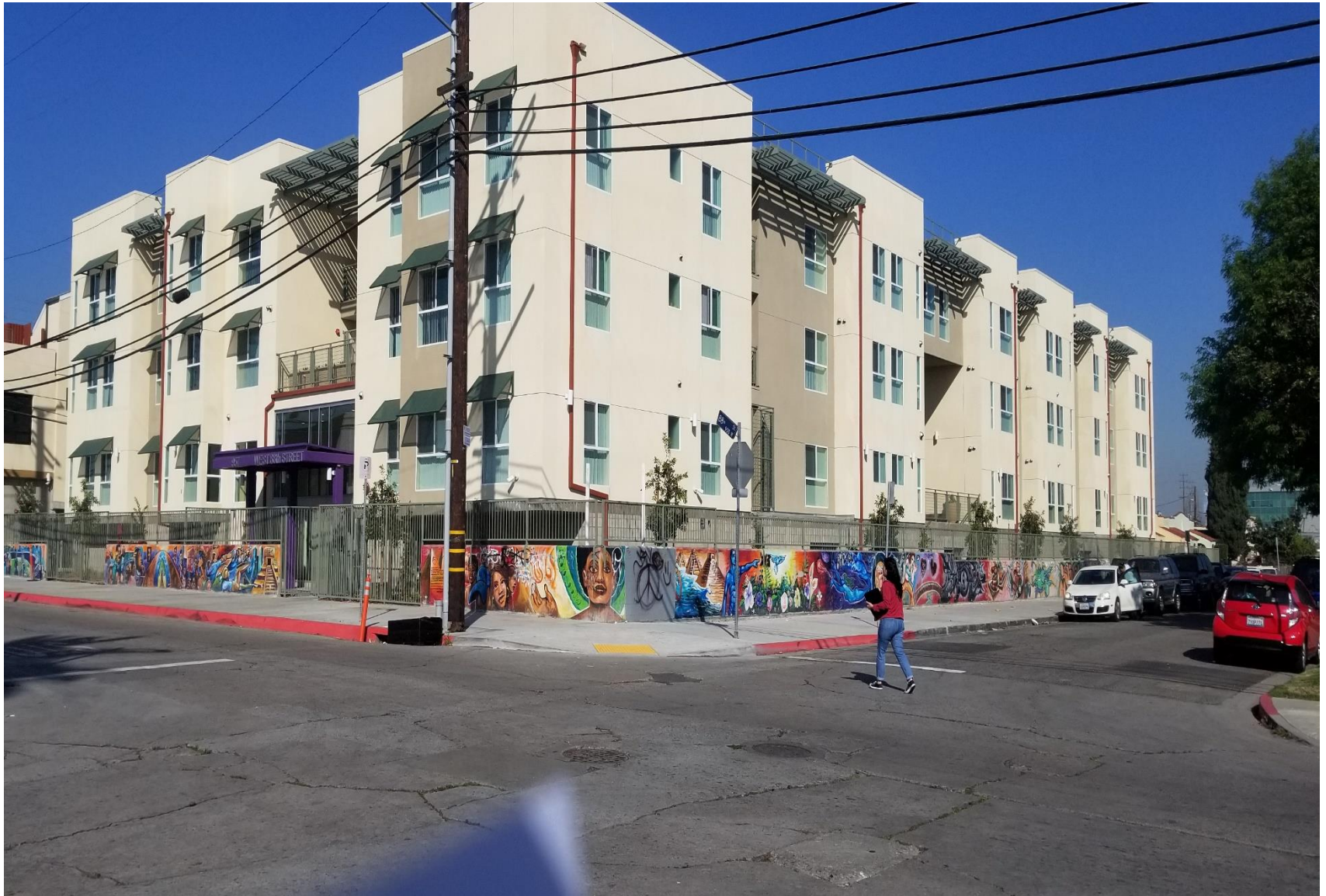
Located at 8707-27 S. Menlo Apts. Bldg 2 residential. View from Menlo & 88 th .
