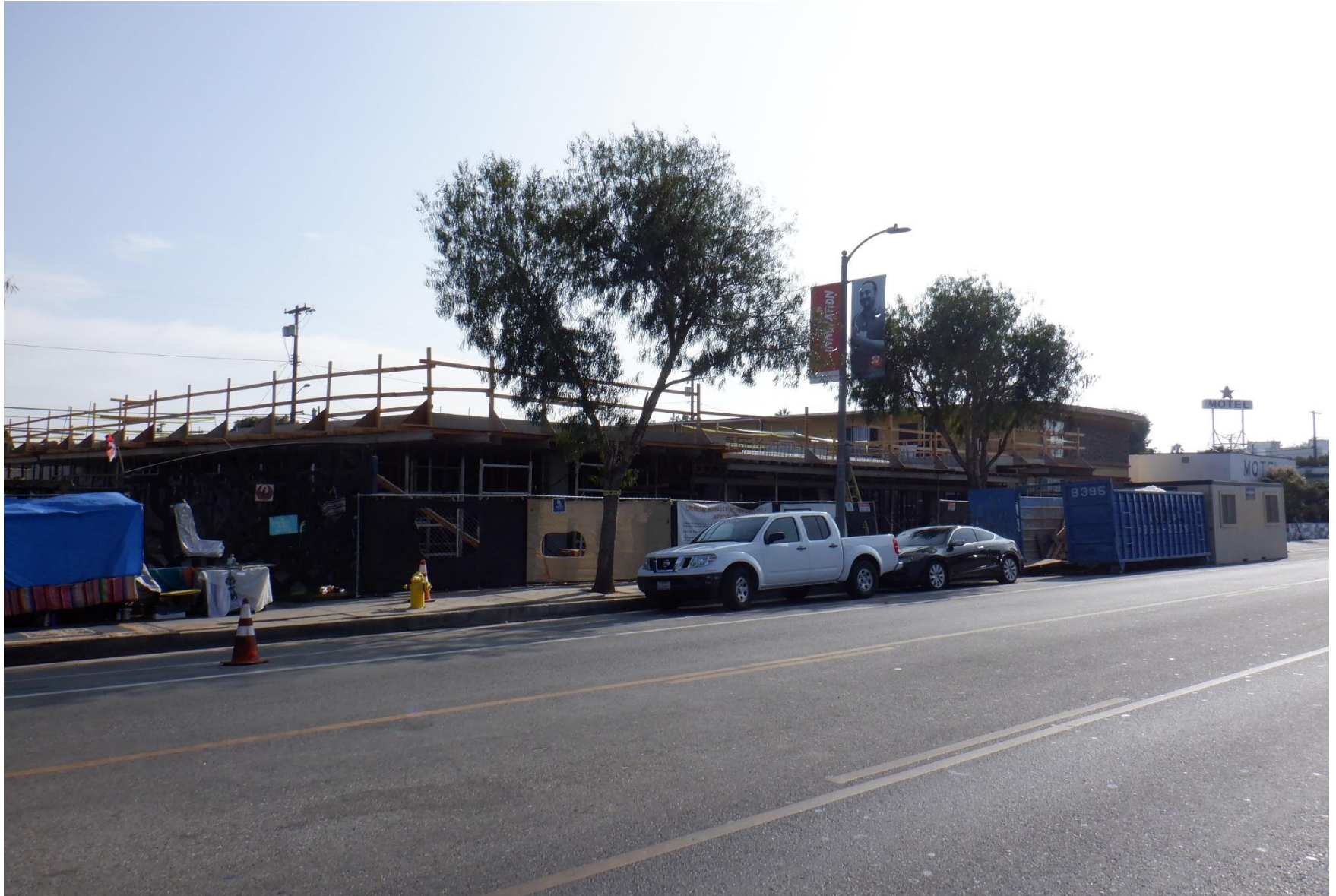
View from across the street at 720 E. Rose Ave.
