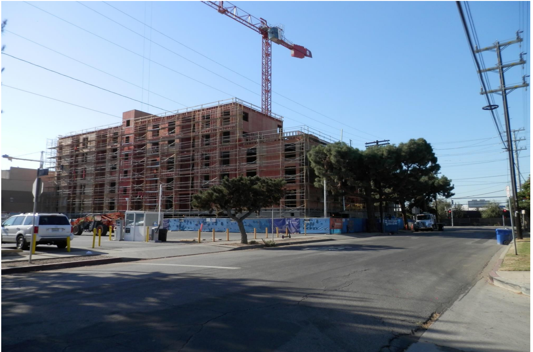
View from corner of Missouri St. & Bundy, on top of second floor open area.
