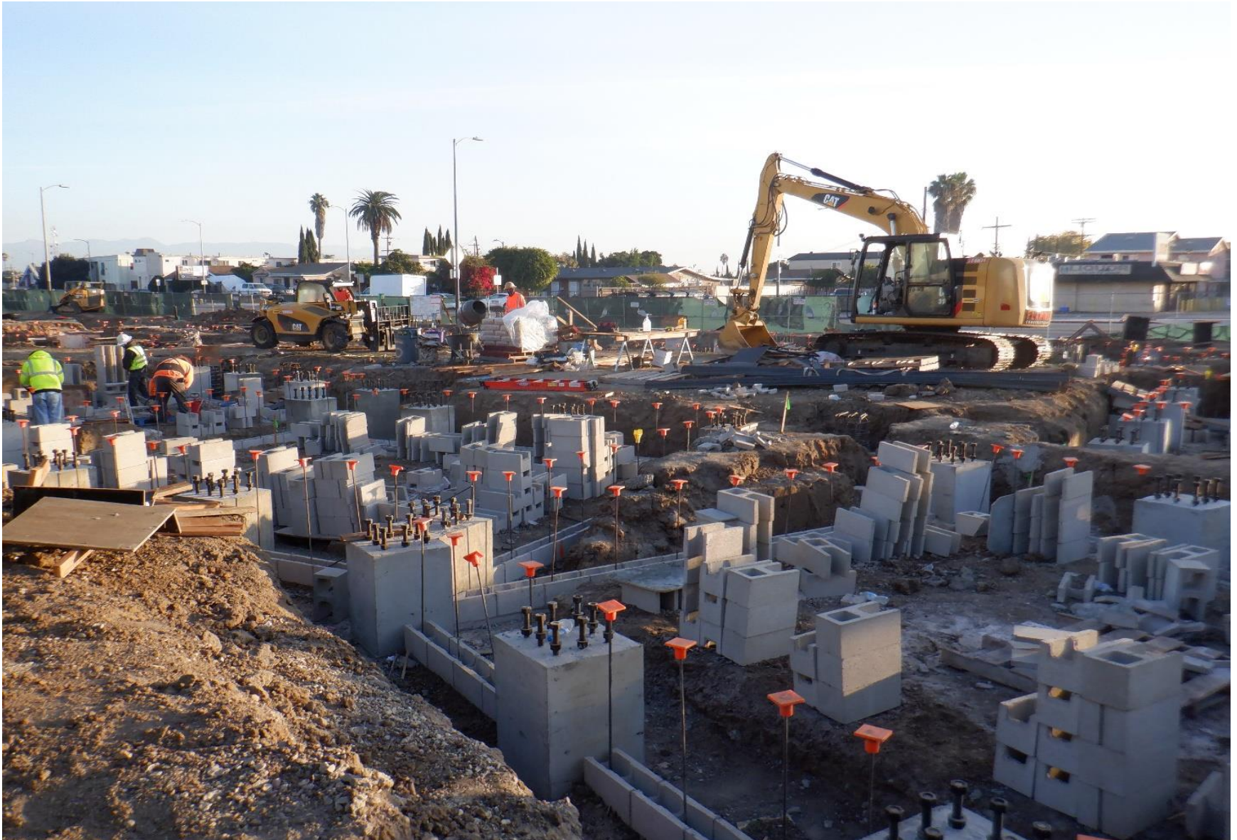
View from inside the fence at 238 W. Imperial Hwy.
