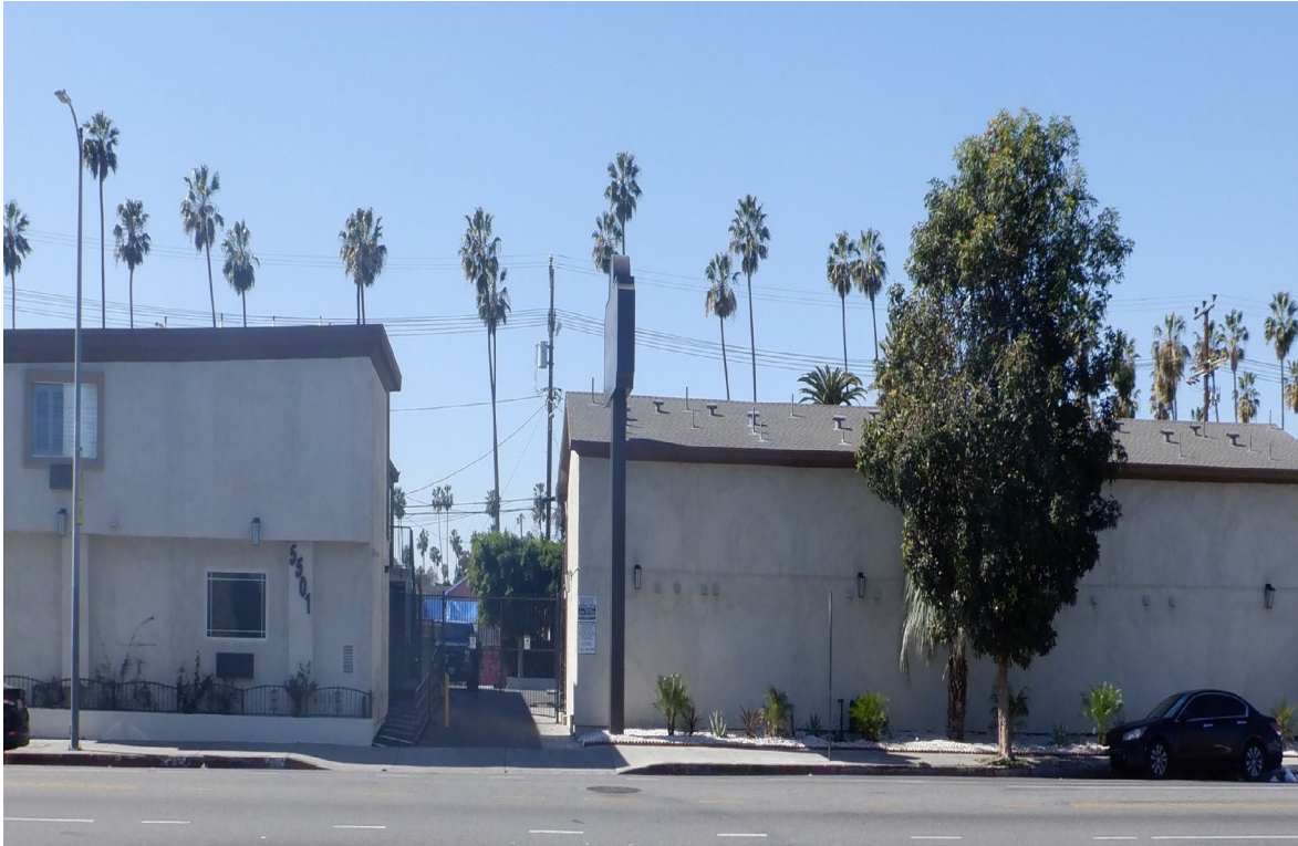
View from across the site at 5501 S. Western Ave.
