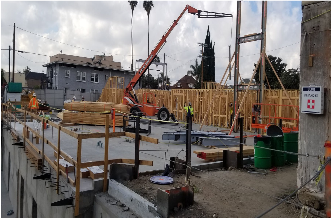
View from inside the fence at 720 W. Washington Blvd.
