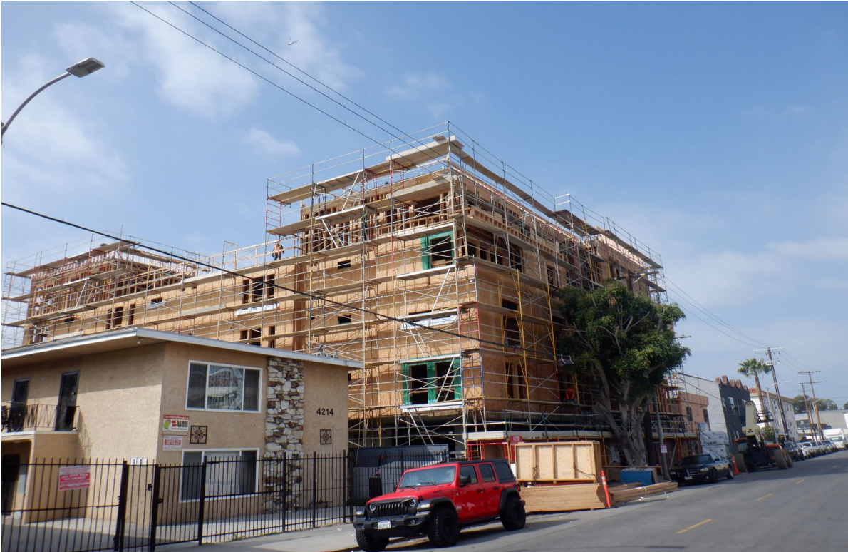
View from across the street at 4220 Montclair St.
