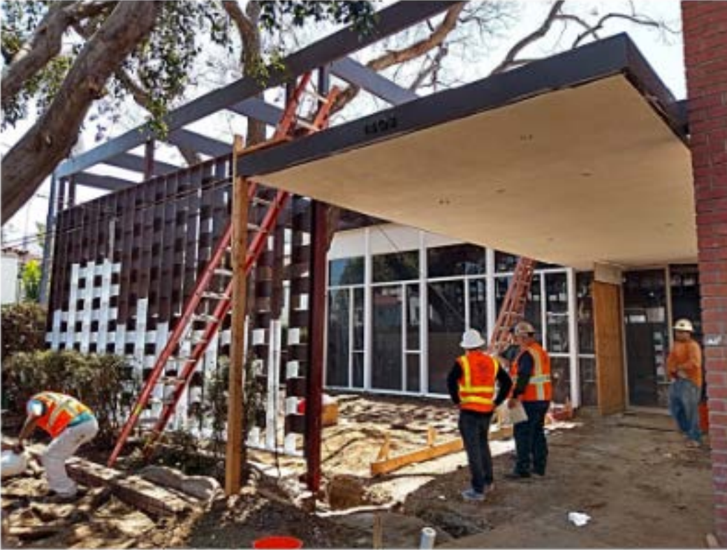
Retrofit and painting of original outdoor structure; trenching
