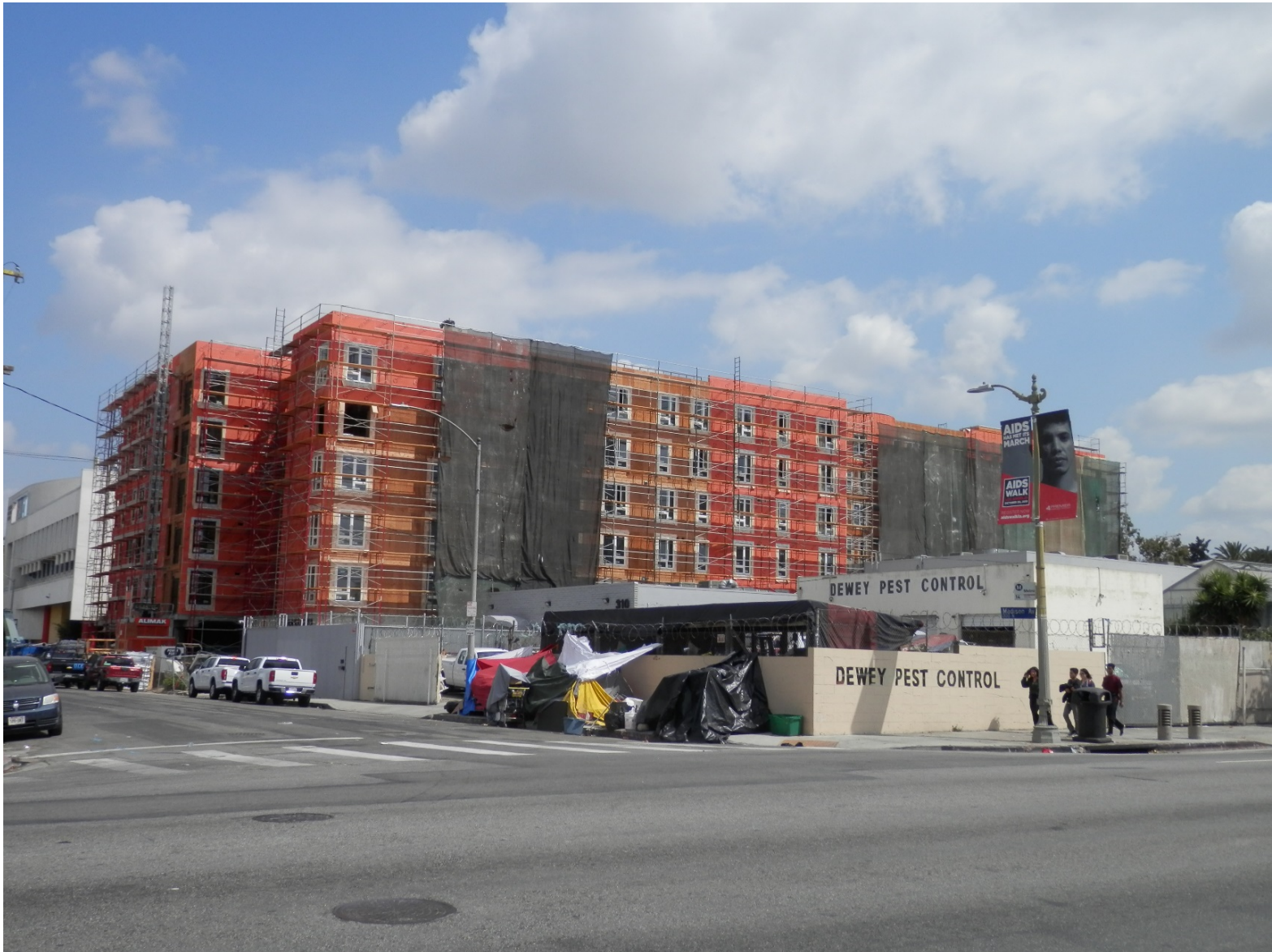
Path Metro Phase 2. View of site at corner of Beverly Blvd & Madison Ave.
