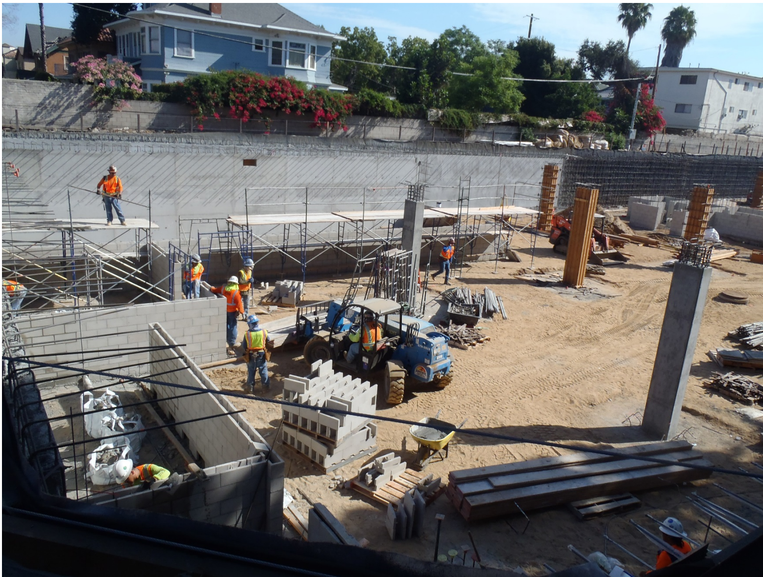
View from just inside the fence at Washington & Gramercy.
