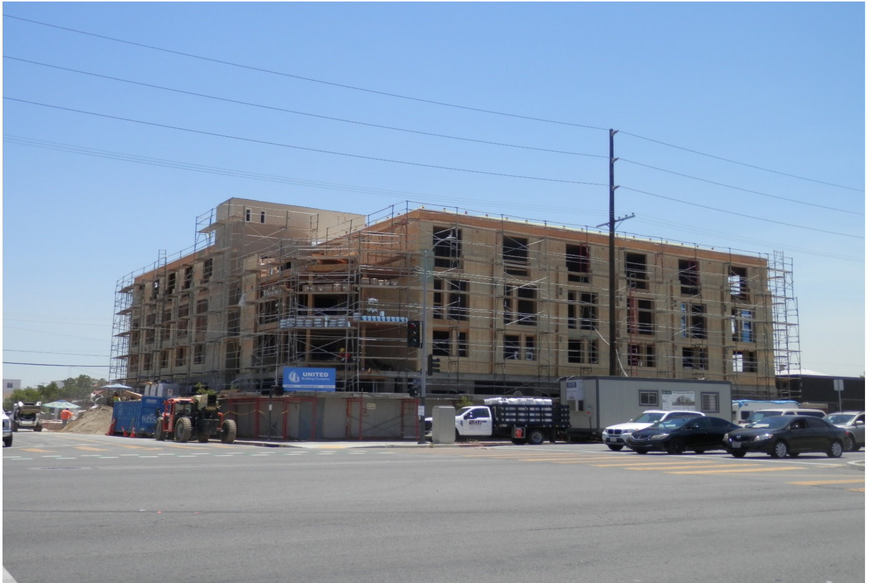
View from across the street at 7600 S Vermont.
