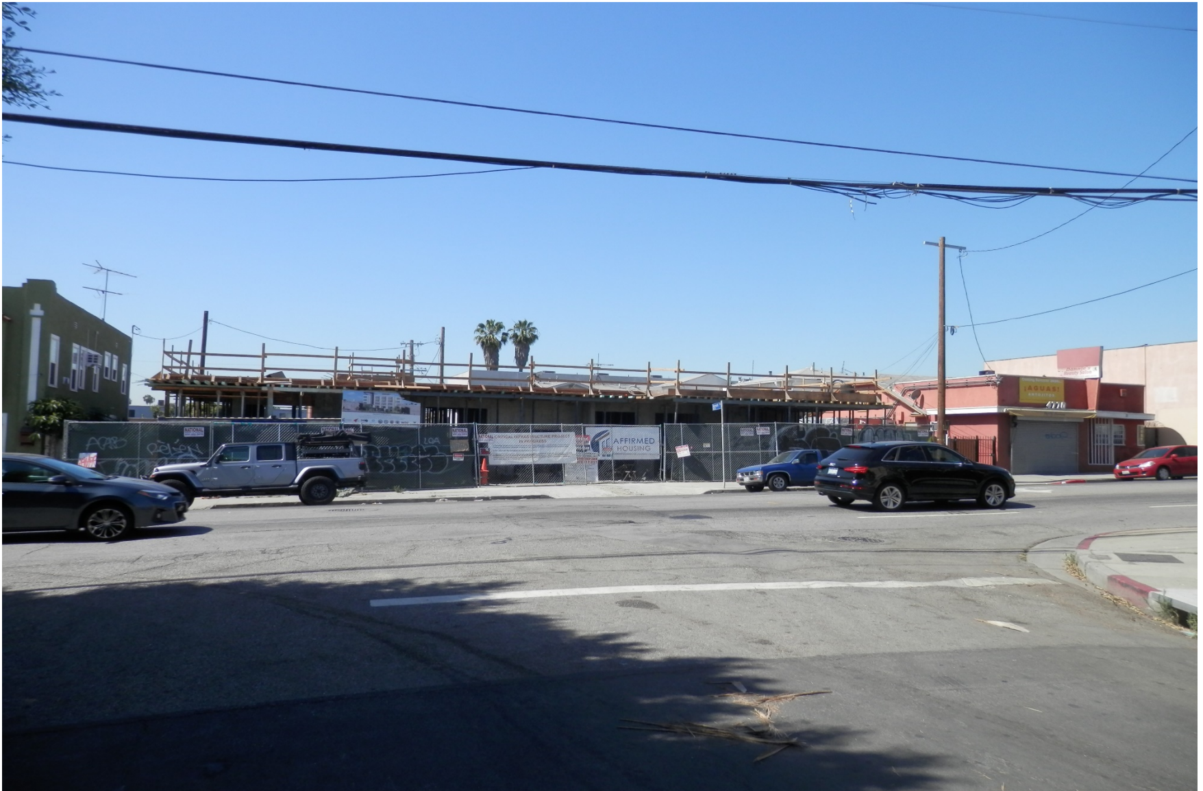
View from across the street at 4760 Melrose Ave.
