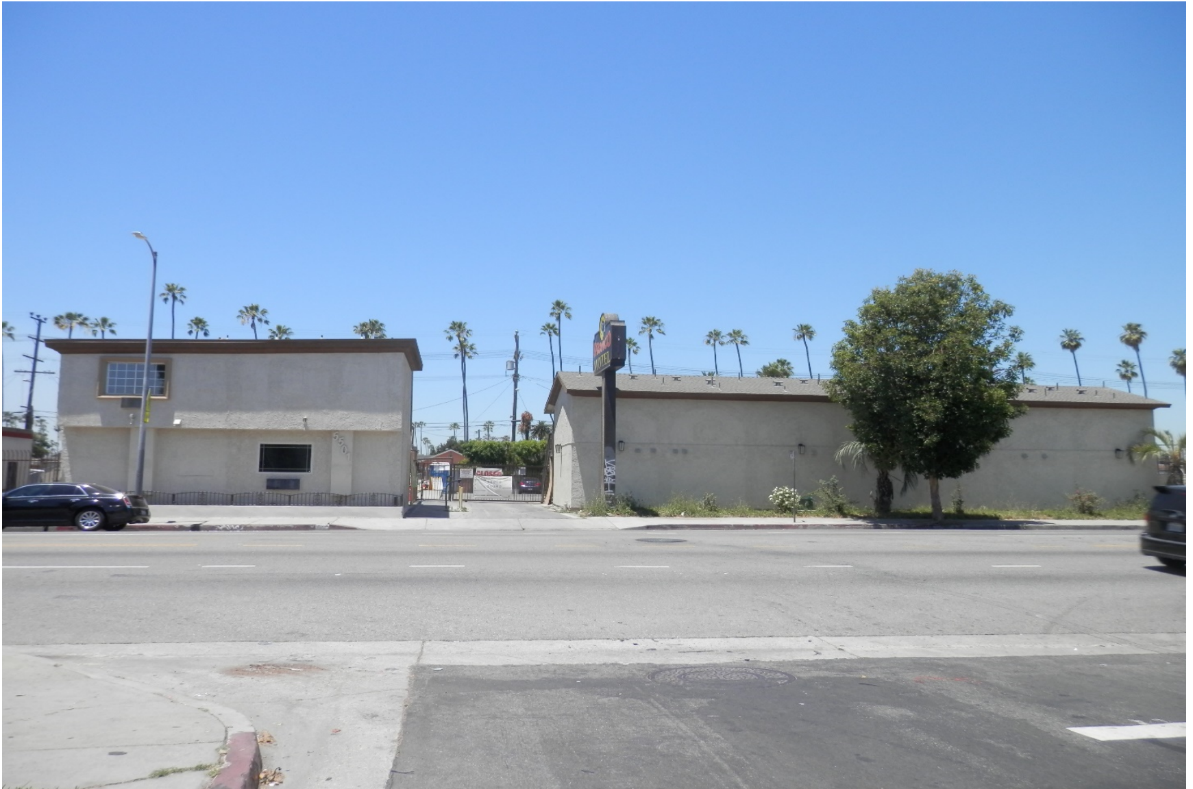
View from across site at 5501 S. Western Ave.
