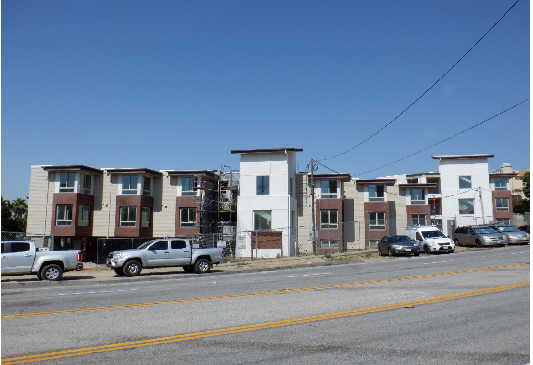
View of the two buildings from front of the site at 13574 Foothill Blvd.
