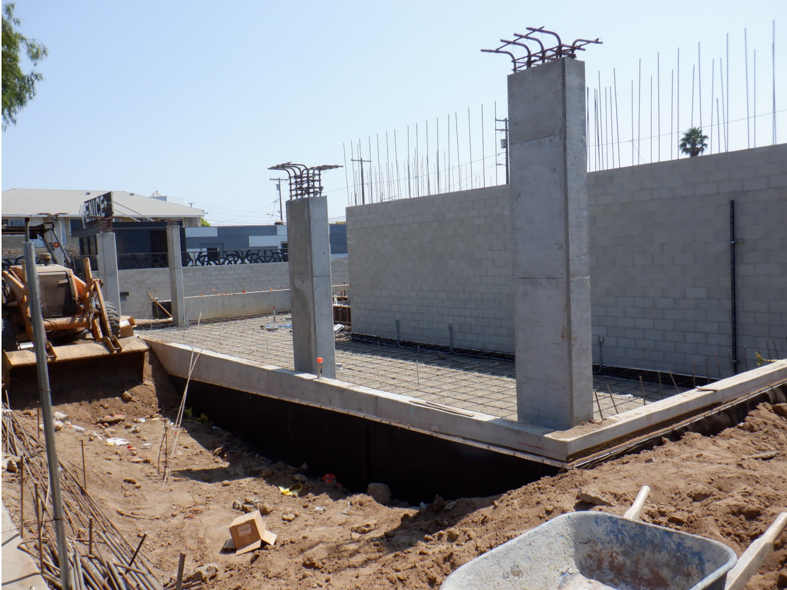
View from inside of the construction fence.
