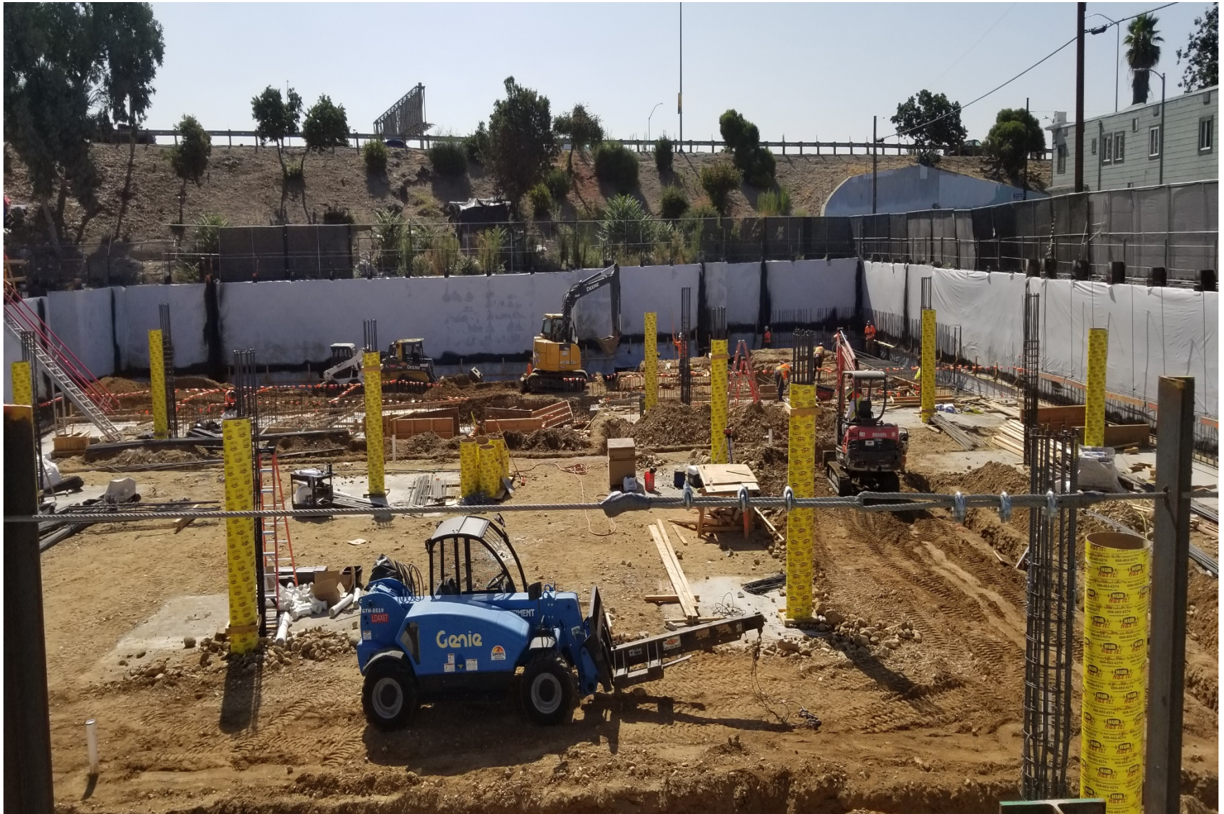
View from just inside the fence at 720 W. Washington Blvd.
