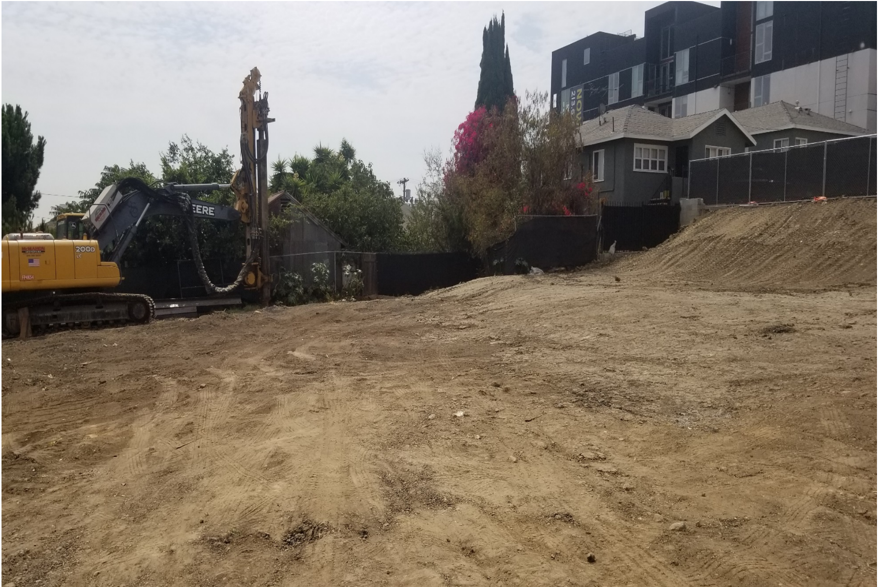
View from just inside the fence at 418 Firmin St.
