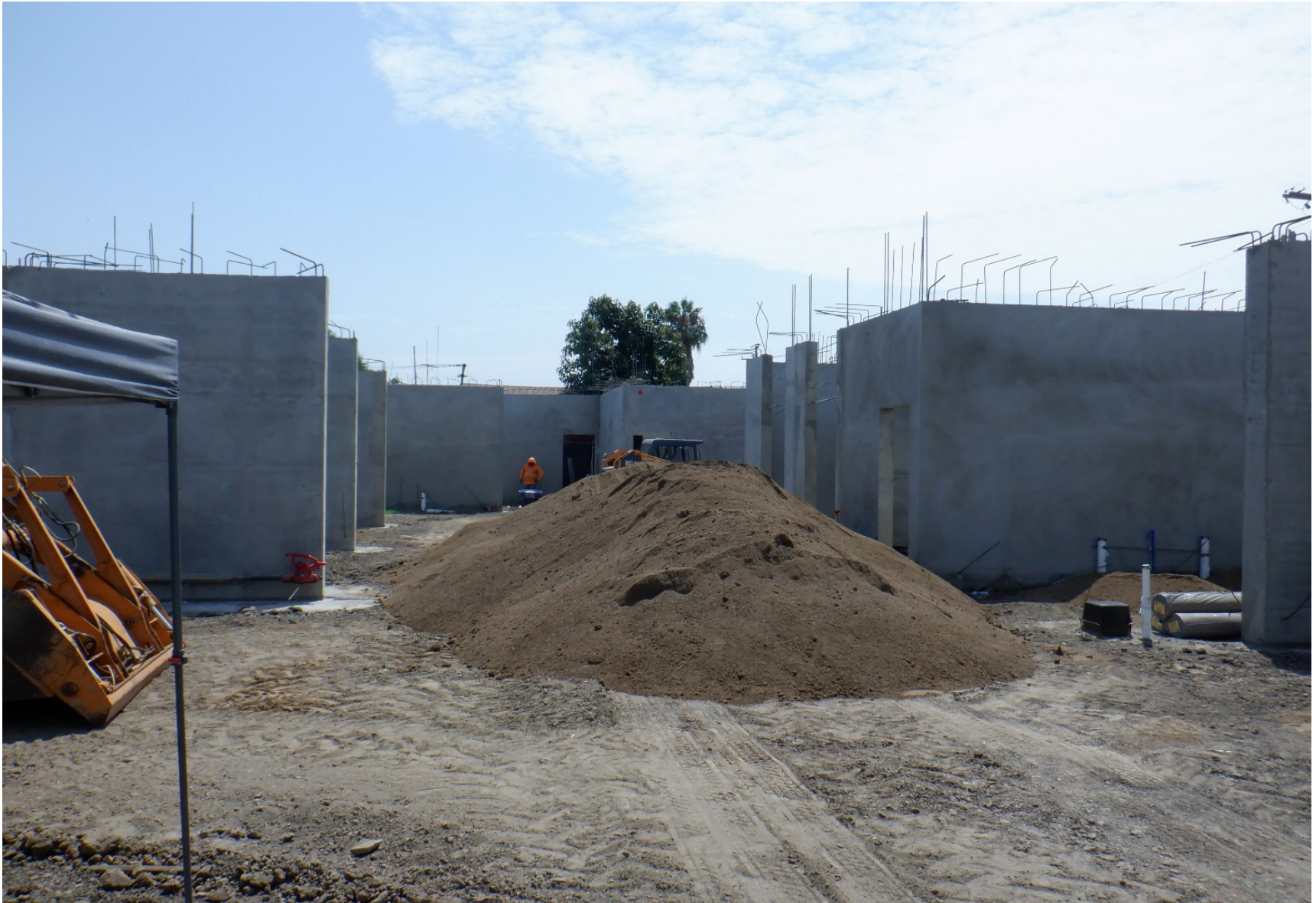
View from just inside the fence at 12003 S. Main St.
